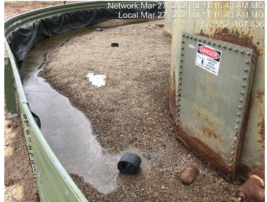
Photo #0849 Trash and unused bull plug in tank containment.
