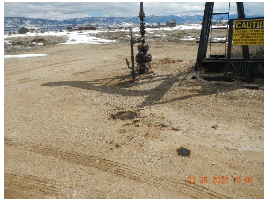
Photo 4. Stained soil at wellhead.
