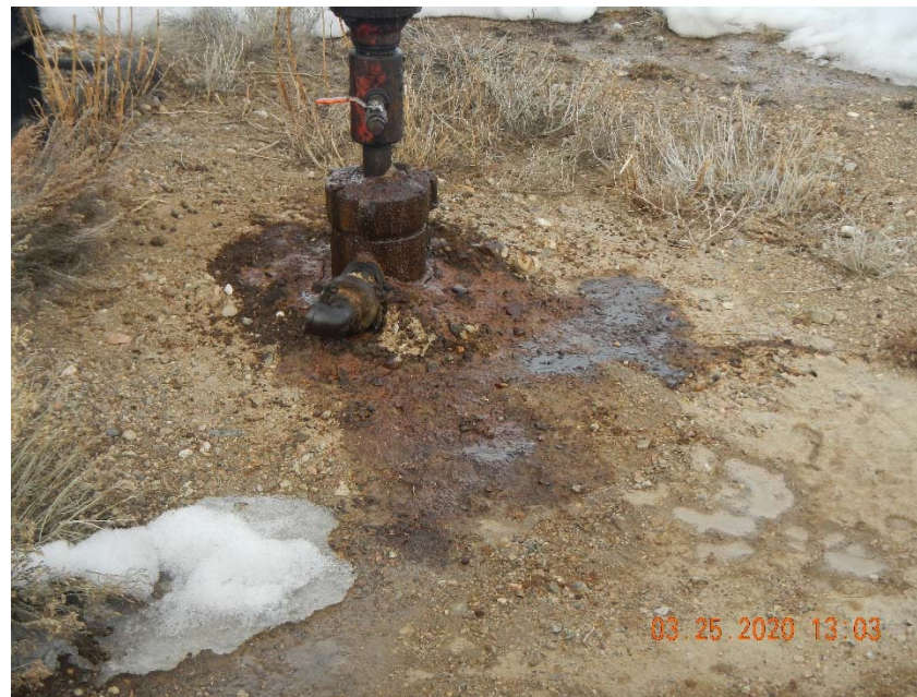
Photo 4. Stained soil at wellhead.
