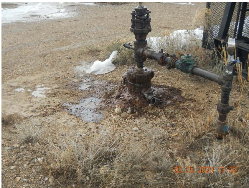
Photo 3. Stained soil at wellhead.
