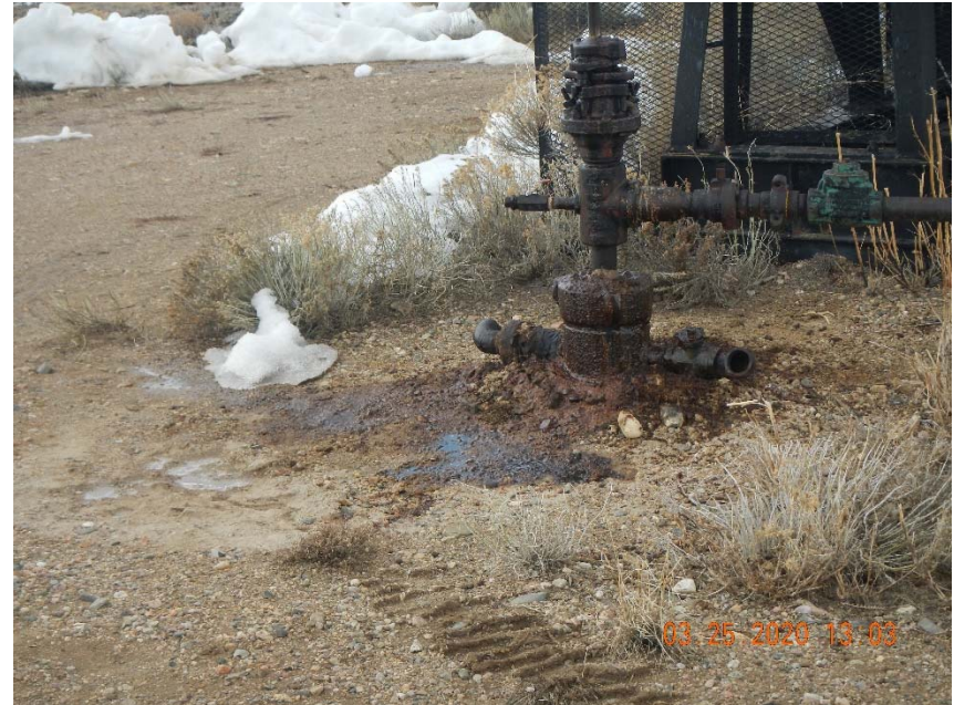
Photo 2. Stained soil at wellhead.
