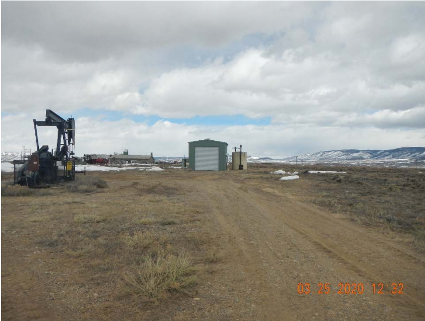
Photo 1. Overview of location taken facing north.
