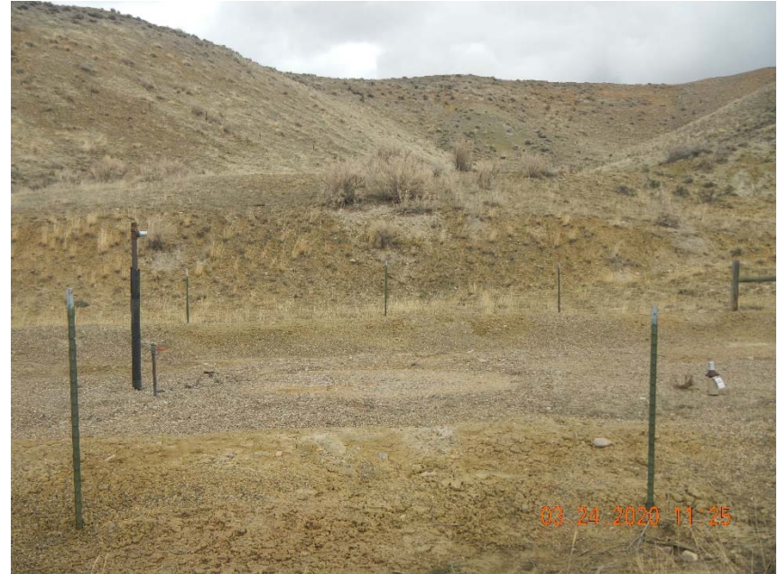
Photo 2. 2 risers on left side of photo not LOTO or marked for abandonment.
