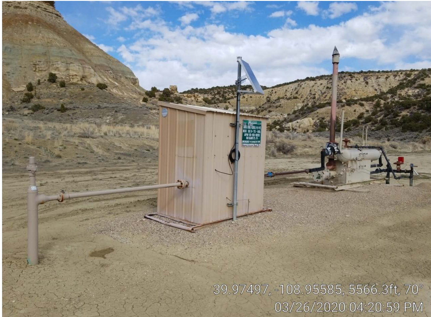
Photo 3. Meter building & separator.
