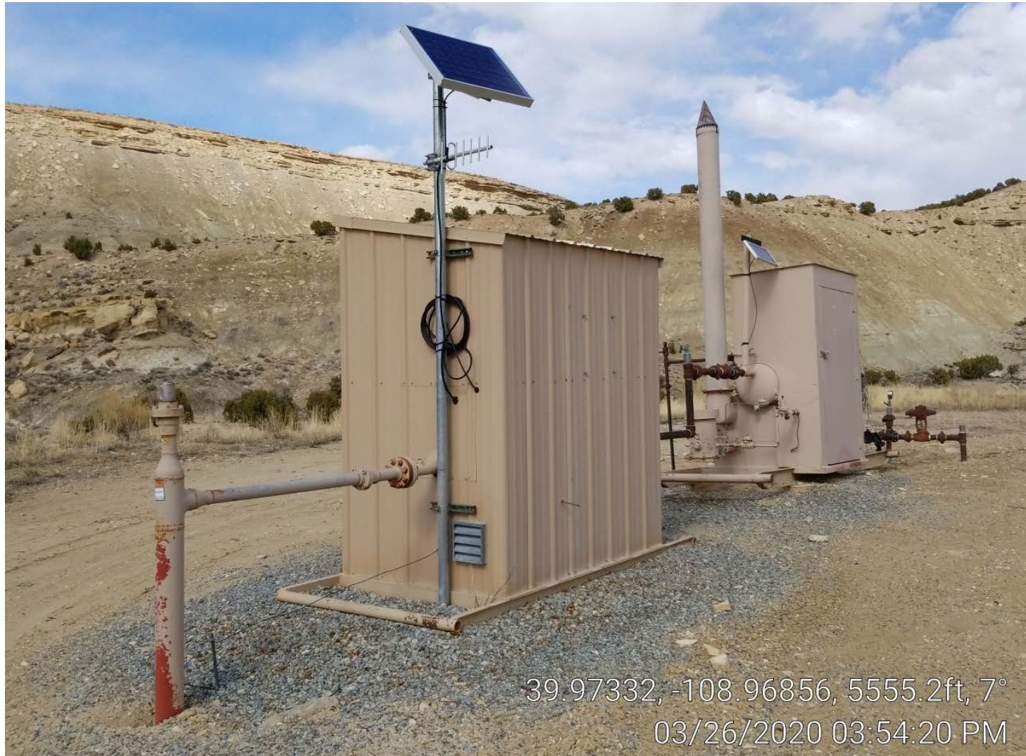
Photo 3. Meter building & separator.
