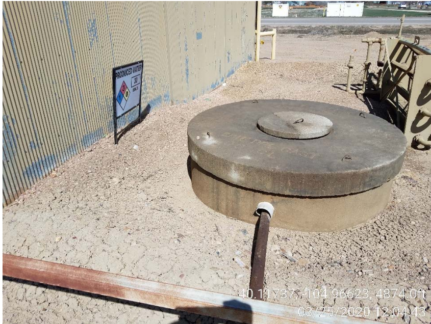
Photo 3 – Buried concrete vessel behind compressor building
