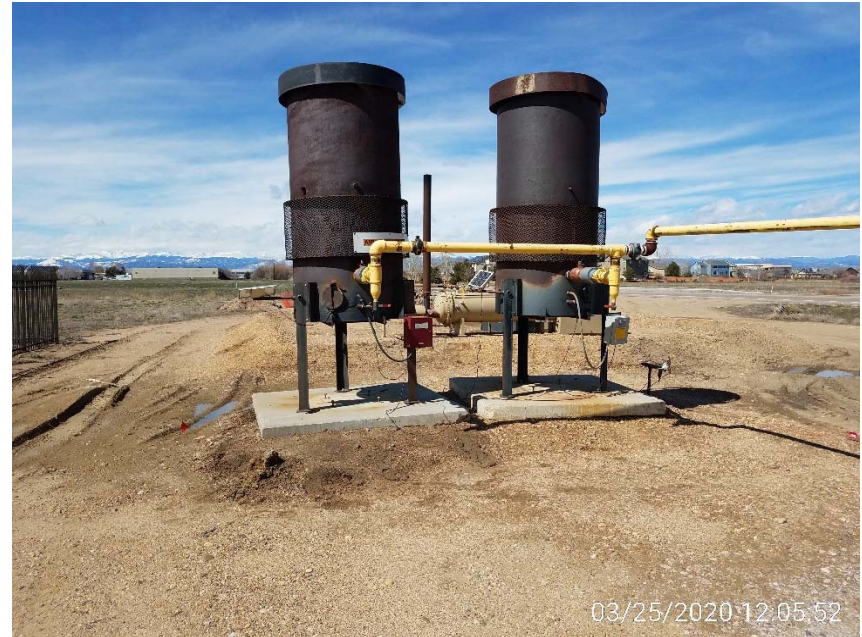
Photo 4 – Emissions Control Device
