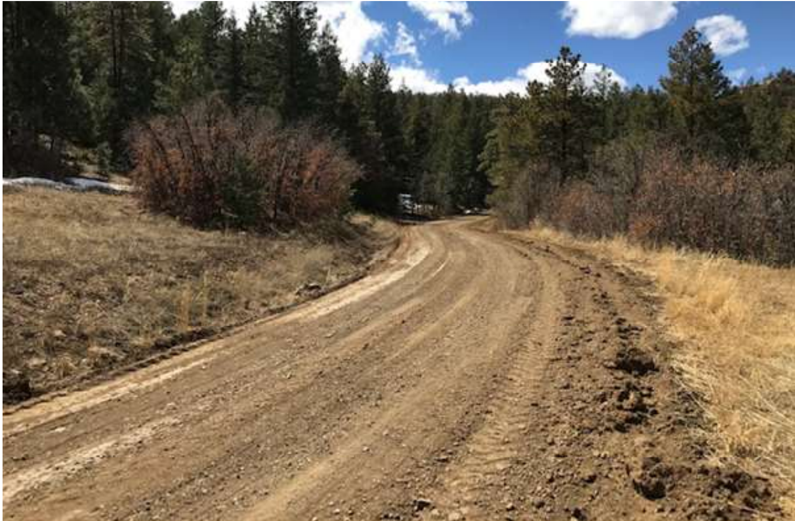
PHOTO 4: FACING SOUTHWEST ALONG THE MAIN LEASE ROAD. THE MAIN LEASE ROAD SURFACE WAS CROWNED TO REMOVE THE TIRE RUTS AND ESTABLISH SHEET FLOW.
