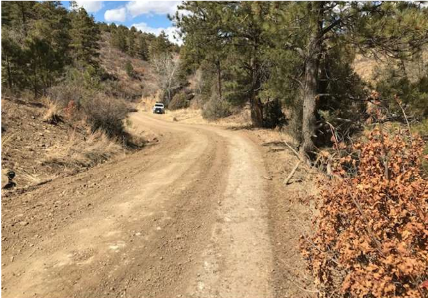
PHOTO 1: FACING SOUTHWEST ALONG THE MAIN LEASE ROAD IN LITTLE BINGHAM CANYON. ONCE THE SOIL DRIED OUT, THE MAIN LEASE ROAD SURFACE WAS CROWNED TO REMOVE THE TIRE RUTS AND ESTABLISH SHEET FLOW.
