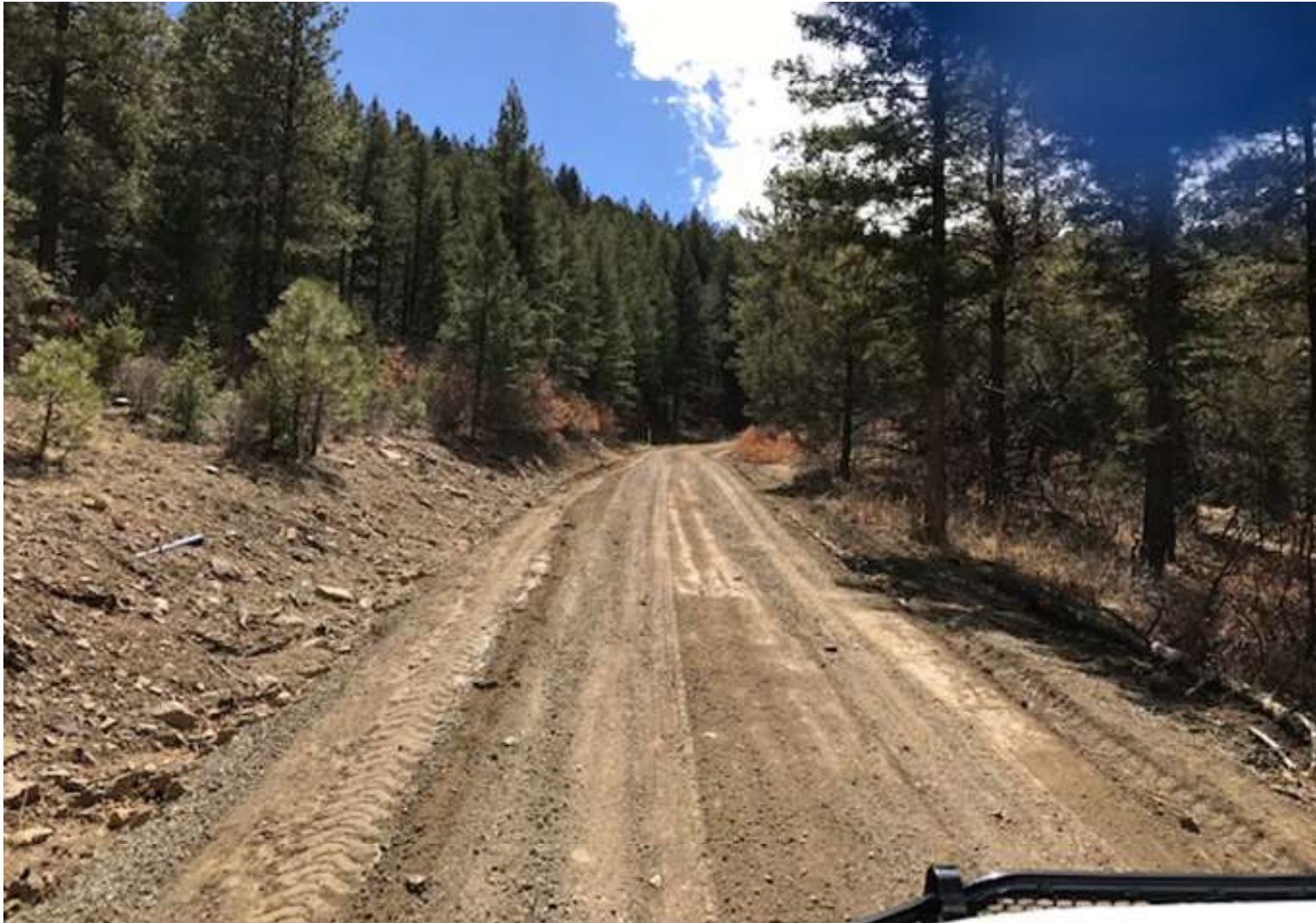
PHOTO 3: FACING SOUTHWEST ALONG THE MAIN LEASE ROAD IN LITTLE BINGHAM CANYON. THE MAIN LEASE ROAD SURFACE WAS CROWNED TO REMOVE THE TIRE RUTS AND ESTABLISH SHEET FLOW.
