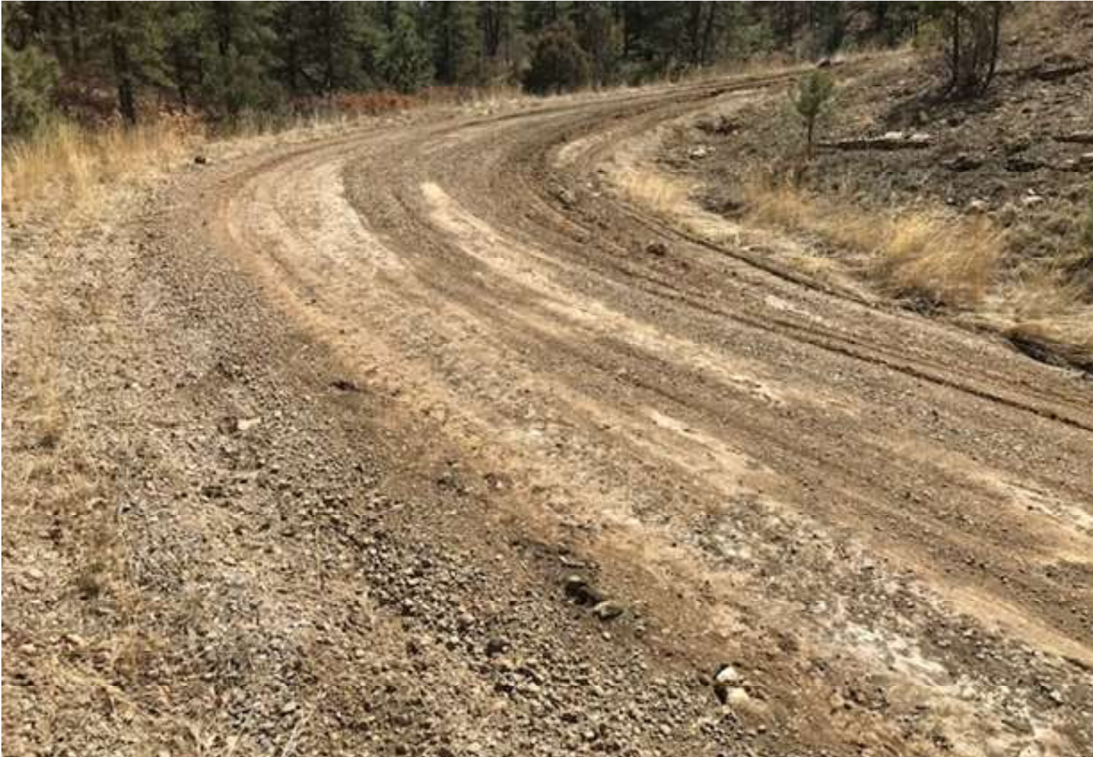
PHOTO 2: FACING SOUTH ALONG THE MAIN LEASE ROAD IN LITTLE BINGHAM CANYON. THE MAIN LEASE ROAD SURFACE WAS CROWNED TO REMOVE THE TIRE RUTS AND ESTABLISH SHEET FLOW.
