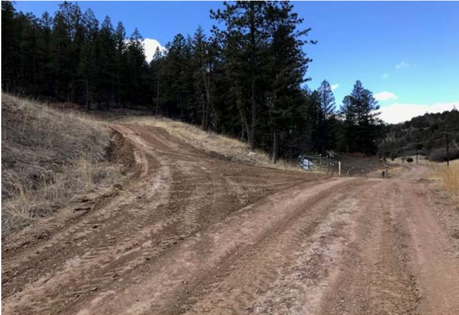
PHOTO 2: FACING SOUTHWEST TOWARD THE ACCESS ROAD TO AC 06-14 WELL PAD. ONCE THE SNOW MELTED AND THE SOIL DRIED OUT, THE ACCESS ROAD SURFACE WAS CROWNED TO REMOVE THE TIRE RUTS AND ESTABLISH SHEET FLOW.
