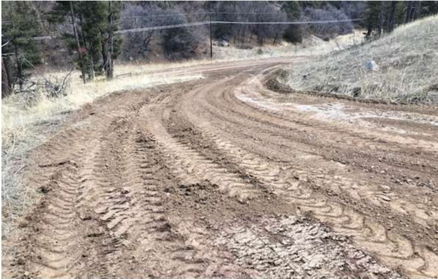
PHOTO 3: FACING BACK TOWARD THE MAIN LEASE ROAD. ONCE THE SNOW MELTED AND THE SOIL DRIED OUT, THE ACCESS ROAD SURFACE WAS CROWNED TO REMOVE THE TIRE RUTS AND ESTABLISH SHEET FLOW.
