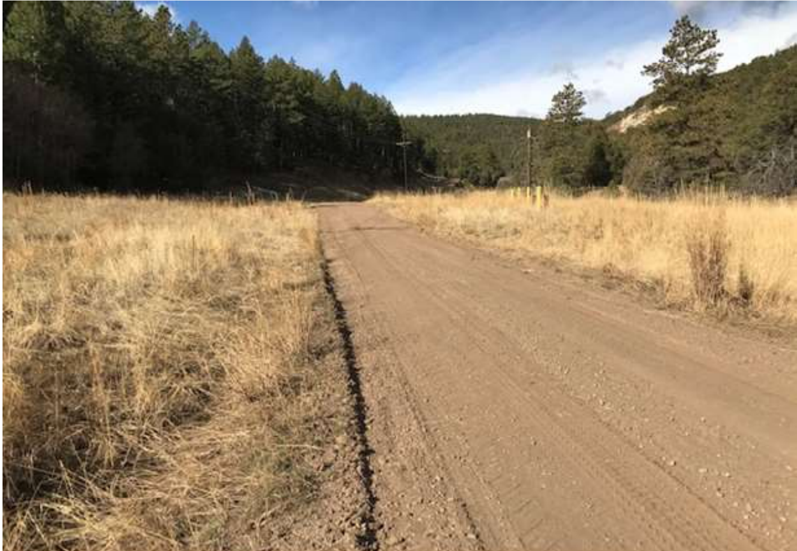
PHOTO 1: FACING WEST ALONG THE MAIN LEASE ROAD IN ALAMOSITO CANYON. THE MAIN LEASE ROAD SURFACE WAS CROWNED TO REMOVE THE TIRE RUTS AND ESTABLISH SHEET FLOW.
