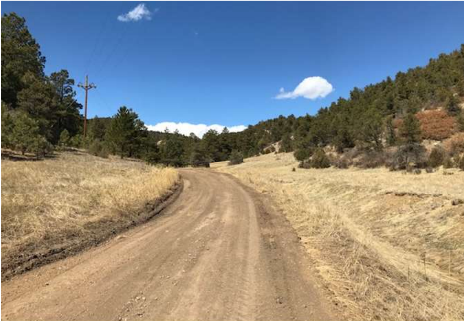
PHOTO 1: FACING NORTHWEST ALONG THE MAIN LEASE ROAD TOWARD THE LOCATION. AFTER THE SNOW MELTED AND THE ROAD SURFACE DRIED, THE MAIN LEASE ROAD SURFACE WAS CROWNED TO REMOVE THE TIRE RUTS AND ESTABLISH SHEET FLOW.
