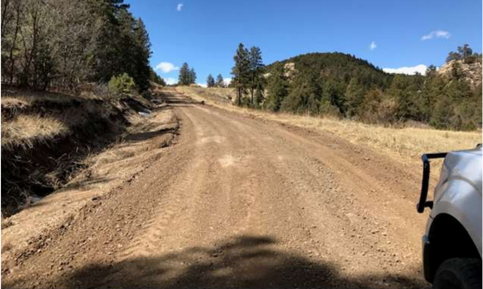
PHOTO 2: FACING NORTHWEST ALONG THE MAIN LEASE ROAD TOWARD THE LOCATION. AFTER THE SNOW MELTED AND THE ROAD SURFACE DRIED, THE MAIN LEASE ROAD SURFACE WAS CROWNED TO REMOVE THE TIRE RUTS AND ESTABLISH SHEET FLOW.
