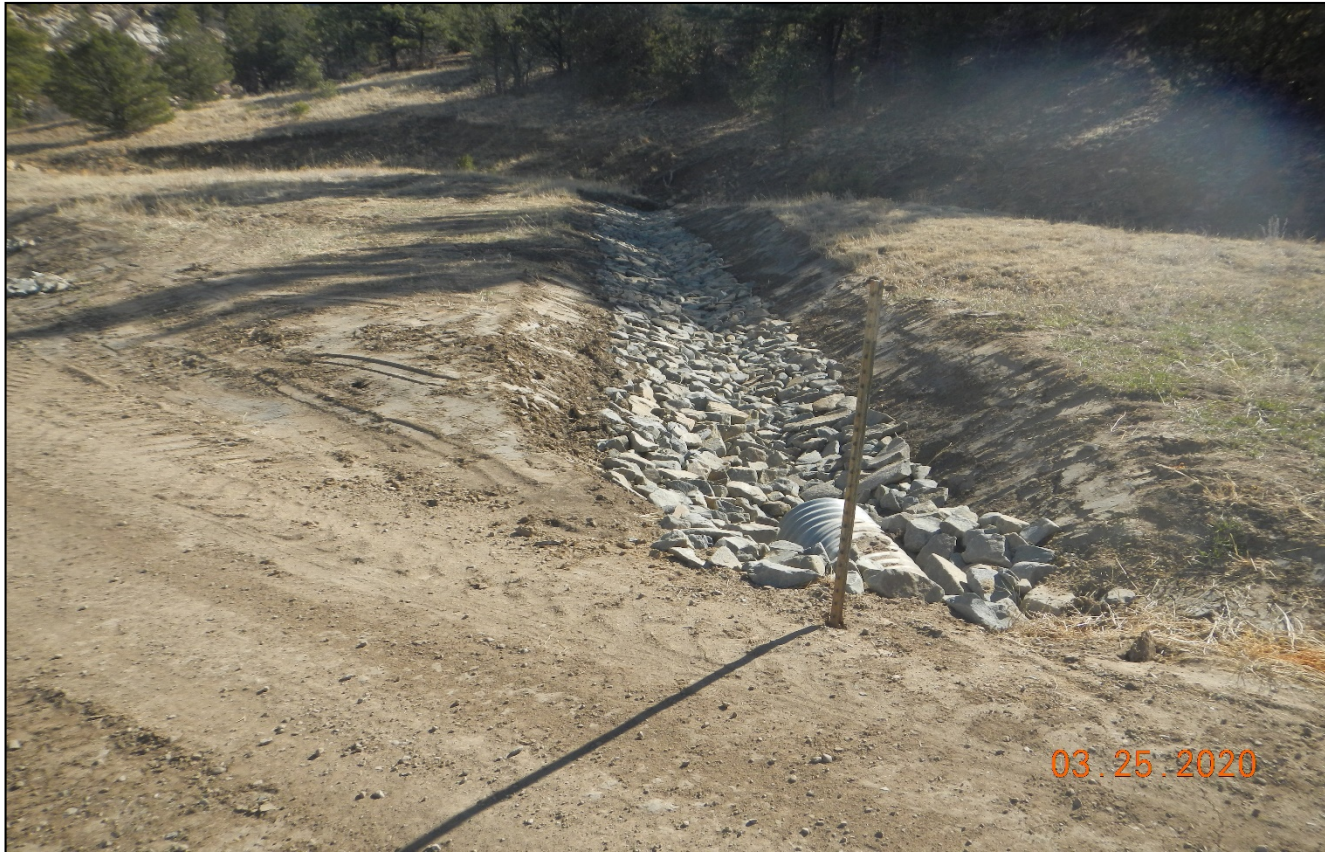
Photo 3. Outlet protection has been installed where erosion was observed at culvert outlet.
