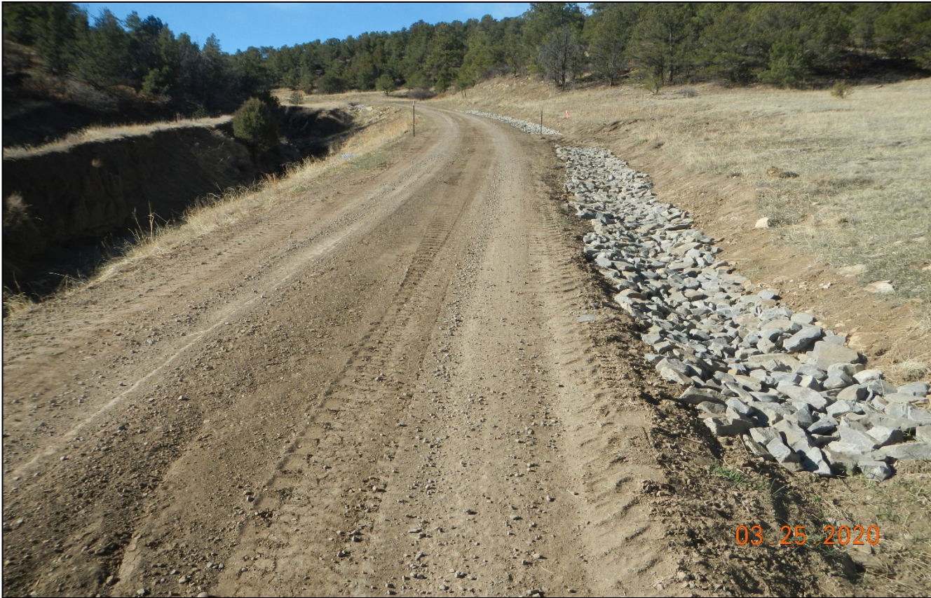
Photo 4. The erosion along the side of the lease road has been repaired and stabilized with rock rip/rap.
