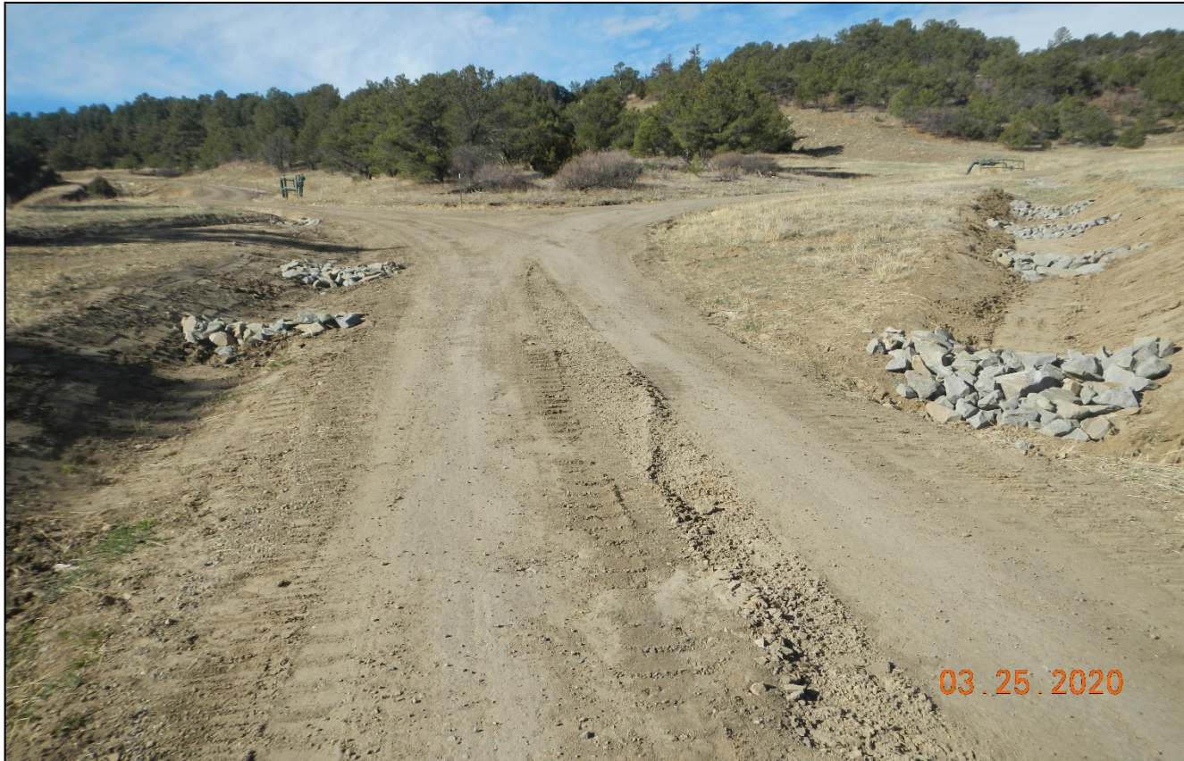
Photo 2. Facing southwest along the main lease road. Rock check dams have been installed along the road in this area.
