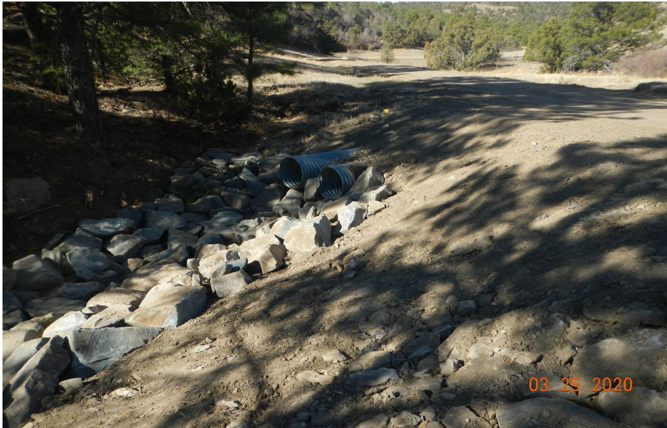
Photo 1. Facing toward culvert outlet along main lease road. Outlet protection has been installed.
