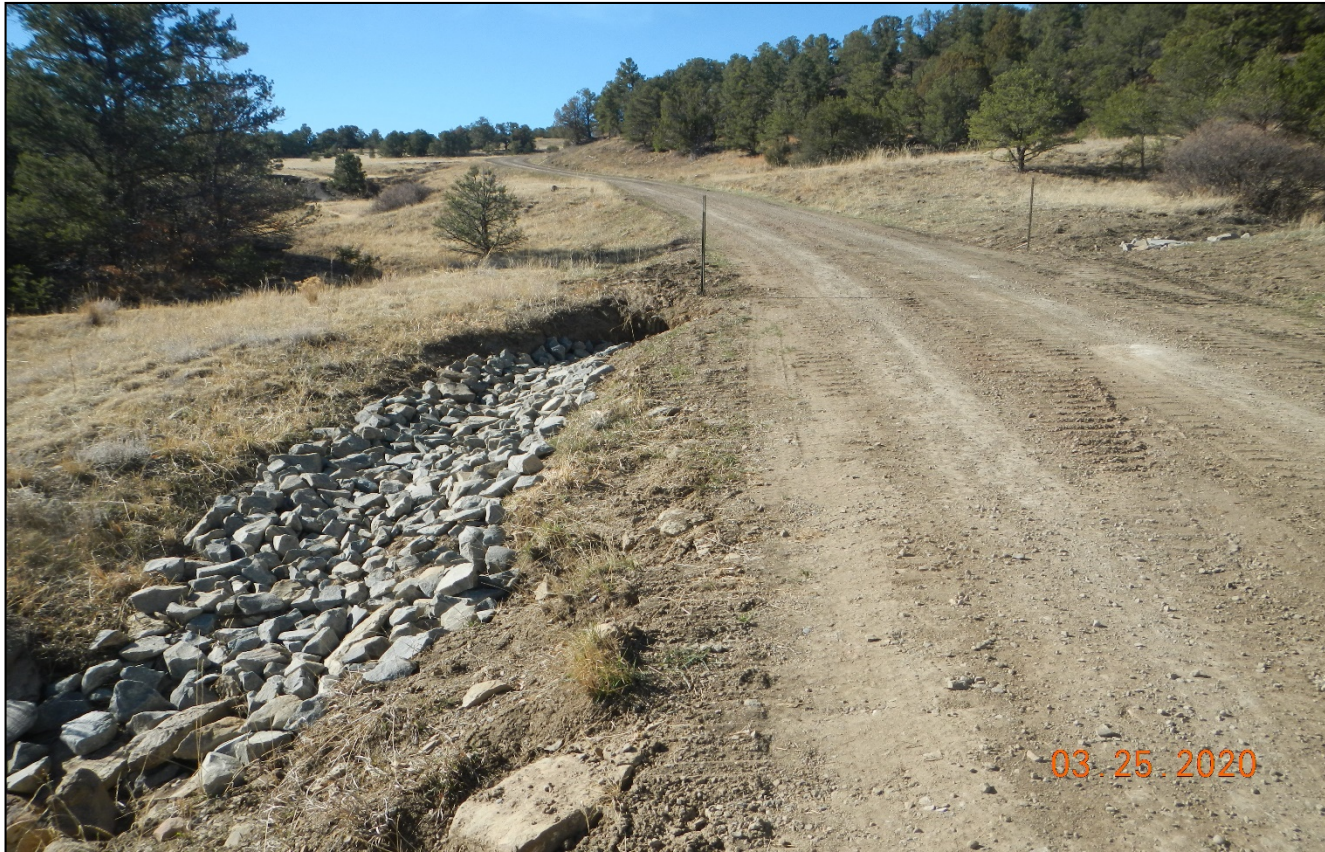
Photo 5. Culvert outlet protection has been installed.
