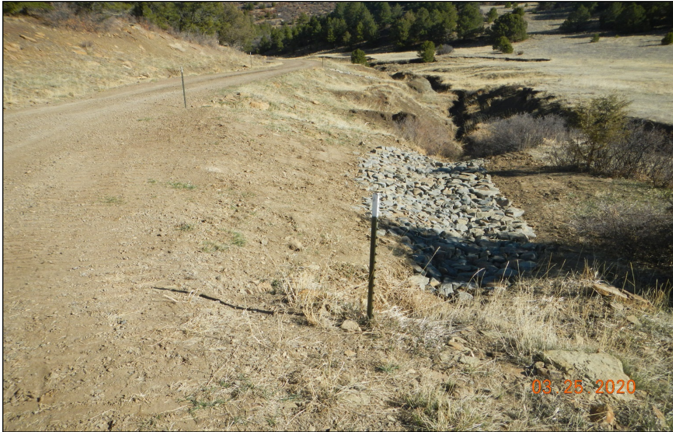
Photo 6. Culvert outlet protection has been installed.
