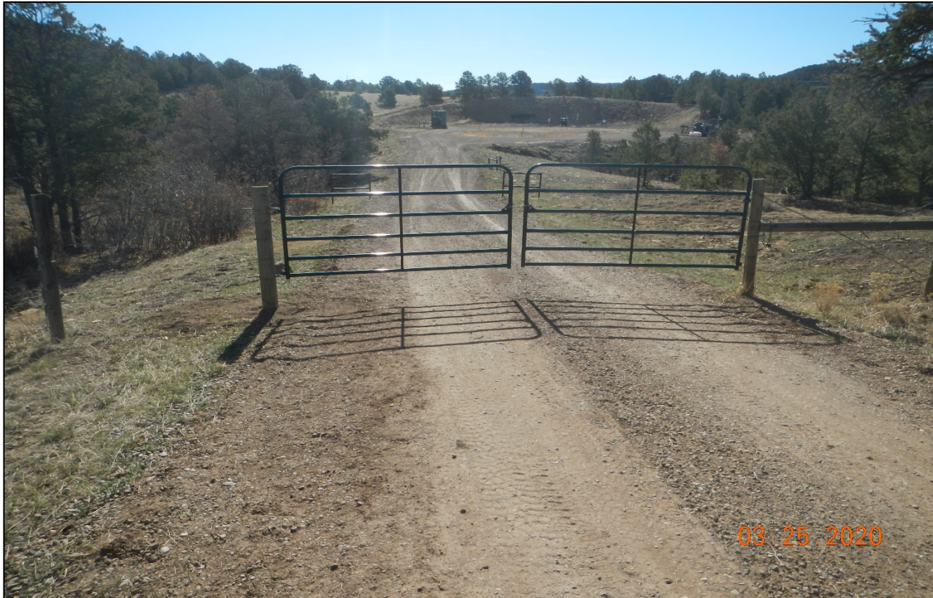
Photo 4. Maintenance has been performed on the gates near the location.
