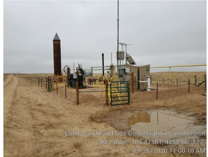
Photo #3 Separator, ECD & Meter Run's
