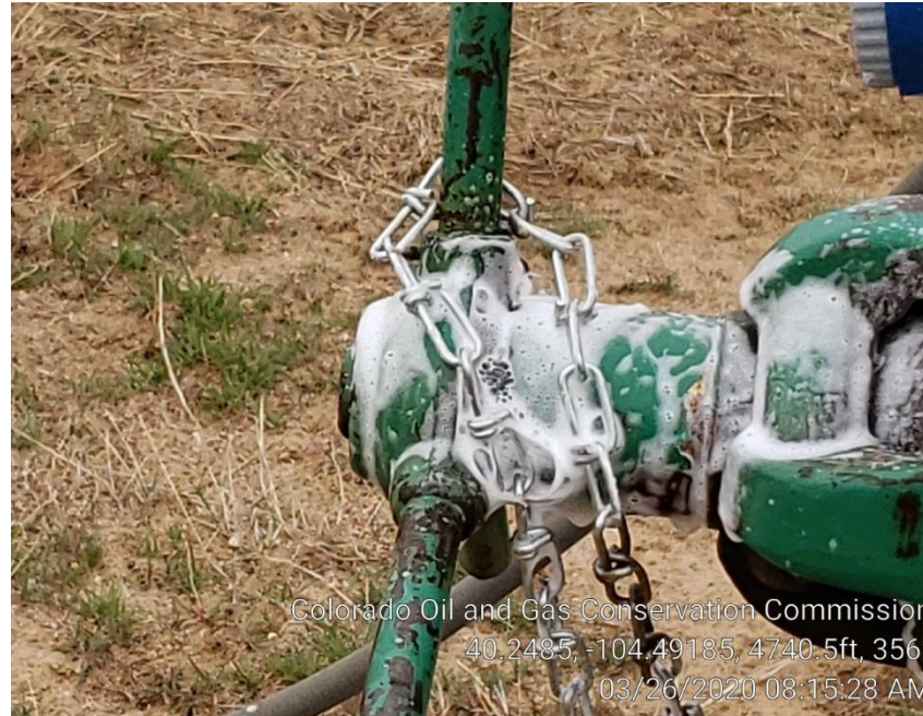
Photo #5 Leaking Master Valve “Gas”
