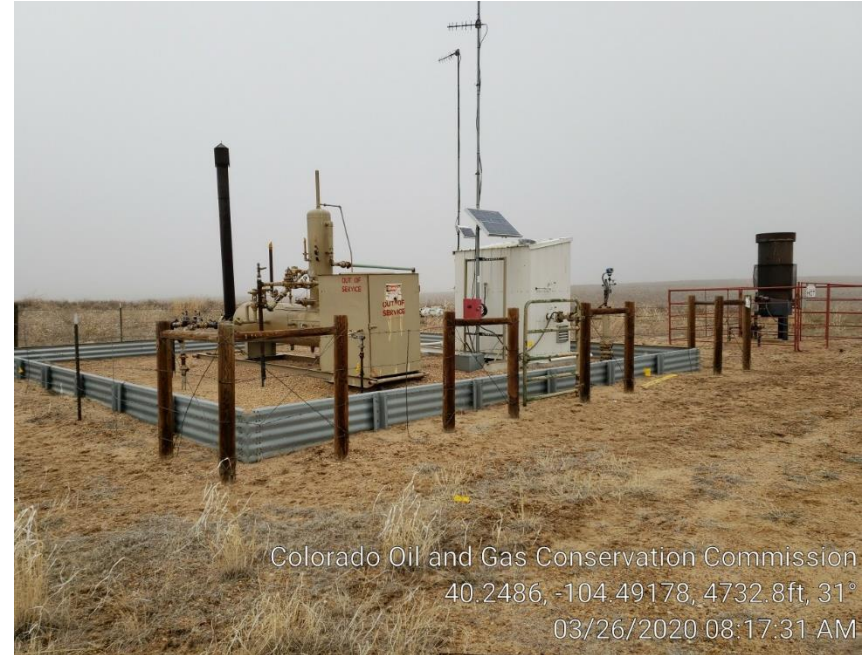
Photo #4 Separator, ECD & Meter Run
