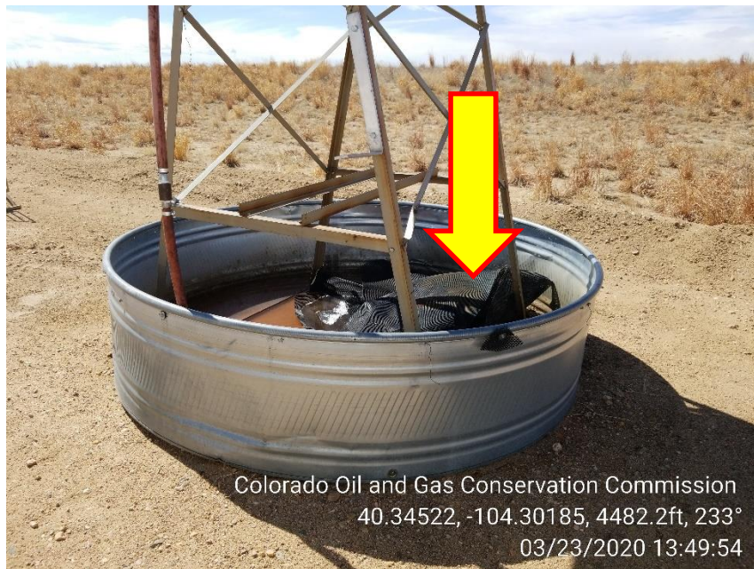
Photo 9 – Containment not covered with Wildlife Netting
