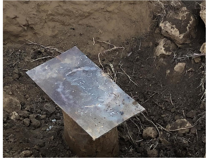
4: Cap plate welded to casing below GL
