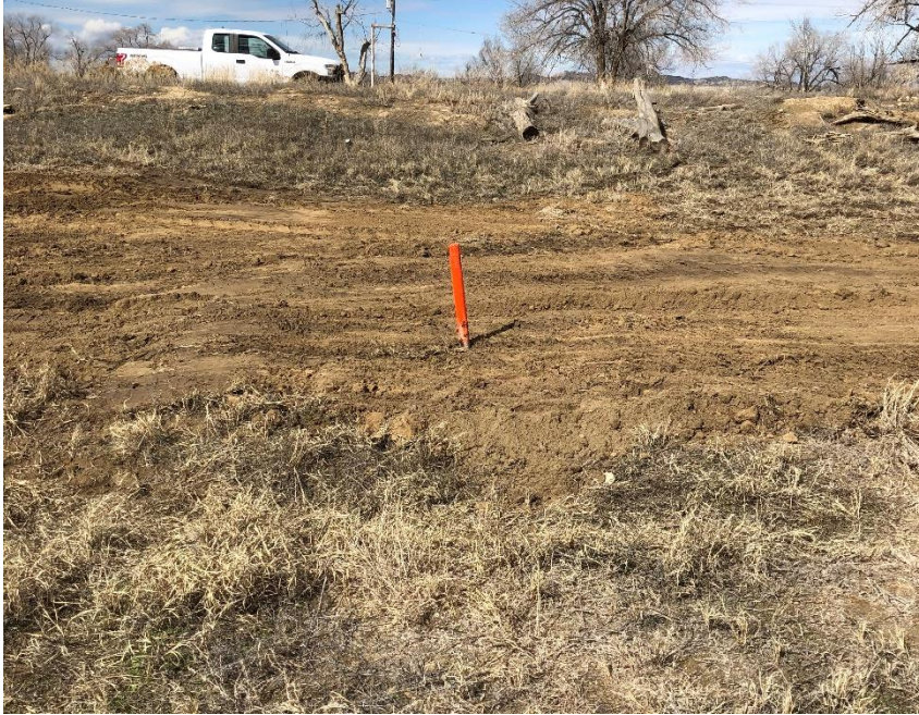
5: Well location filled in and marked with orange post for GPS reading
