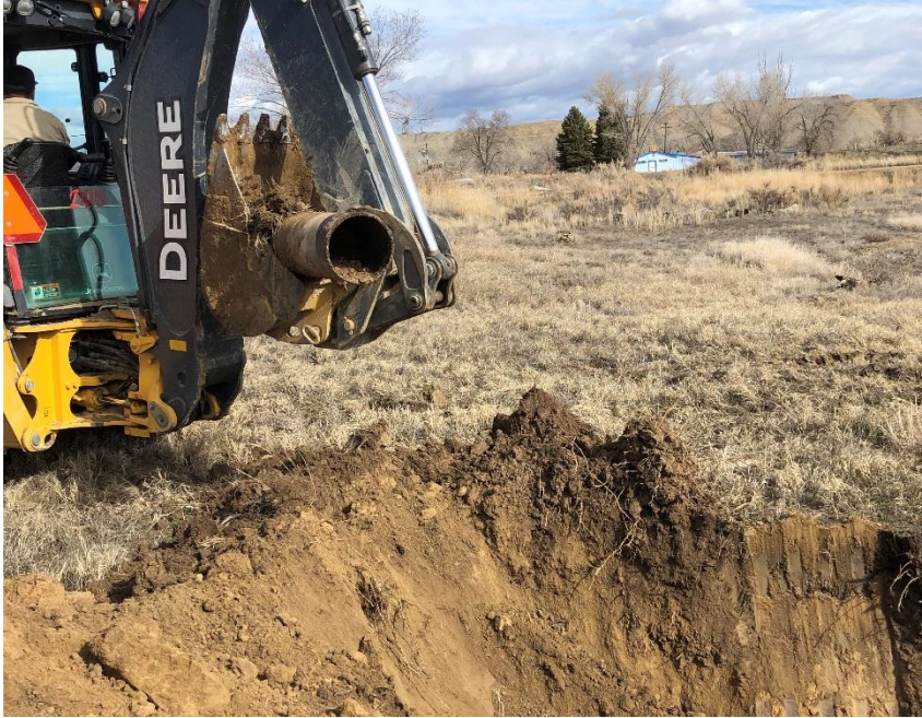
1: Digging out below GL on W H Coltharp 3 and removing cut off casing
