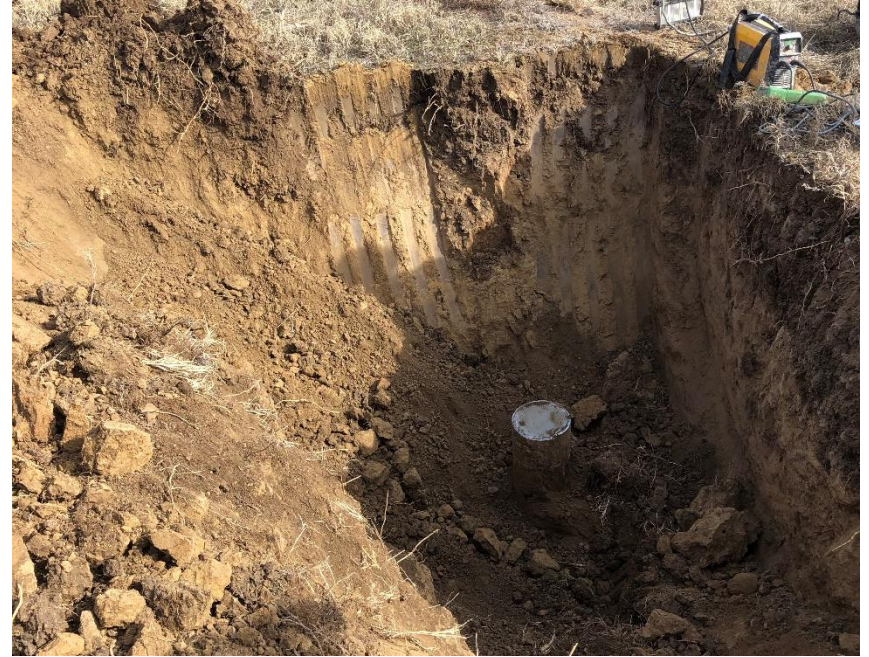
2: Casing cut below GL with cement visible in casing at surface
