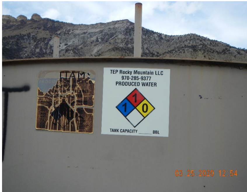
Capacity faded on tank label. (Out of service)
