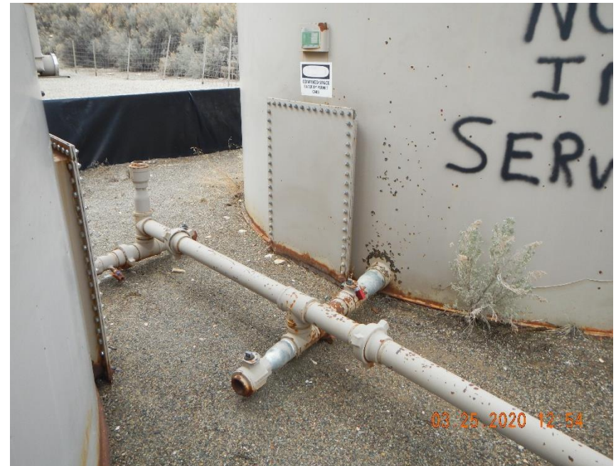
Out of service tank plumbed into other tanks. Master valve shut and locked with padlock.
