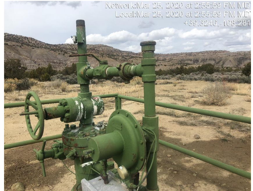
Photo #0840 Multiple flow line risers not LO/TO.
