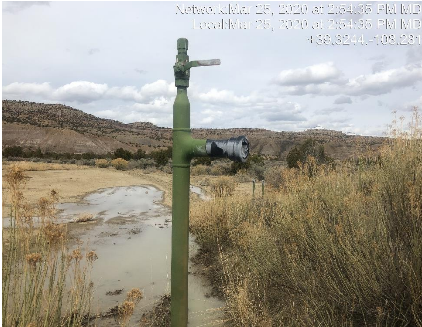
Photo #0837 Multiple flow line risers not LO/TO.
