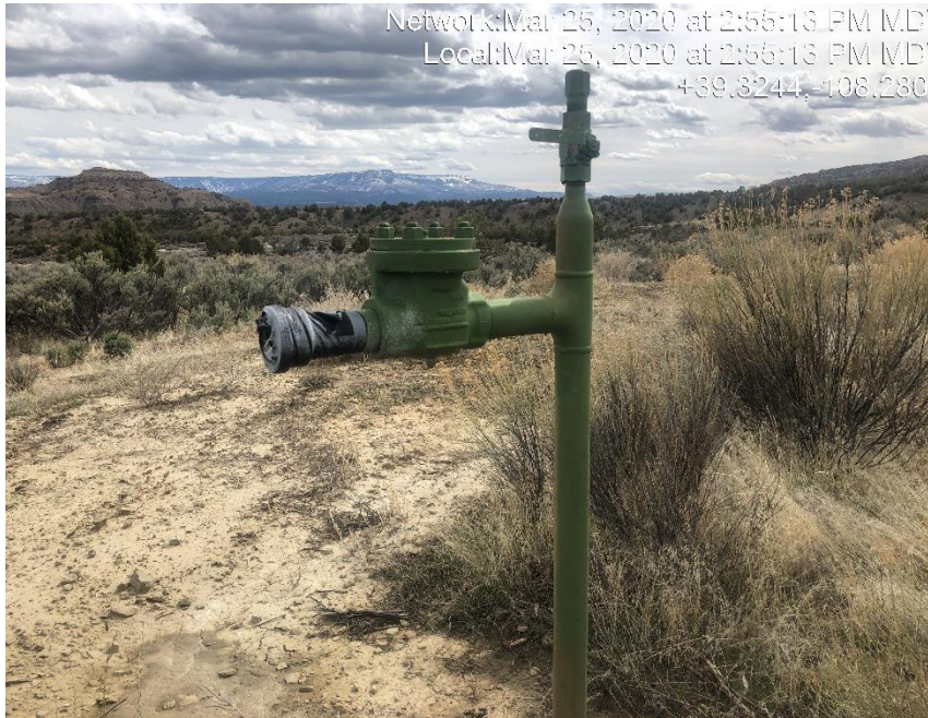
Photo #0839 Multiple flow line risers not LO/TO.
