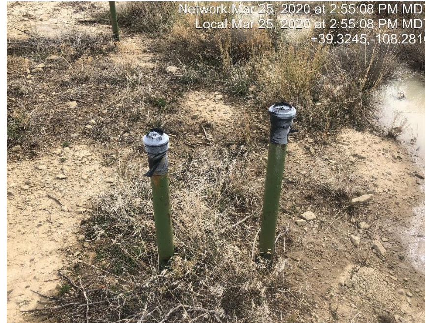
Photo #0838 Multiple flow line risers not LO/TO.
