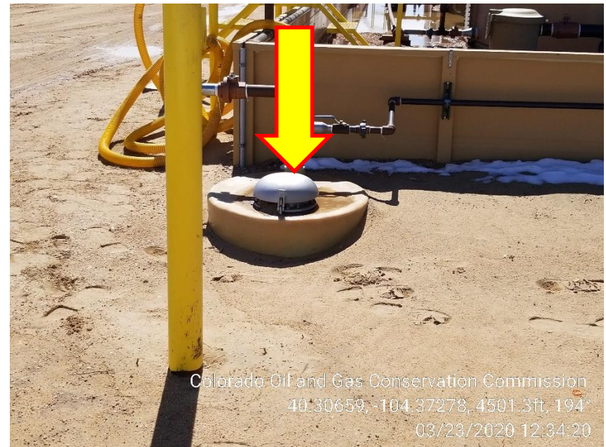
Photo 24 – Fiberglass Vault at NE corner of Tank Berm missing Signage.
