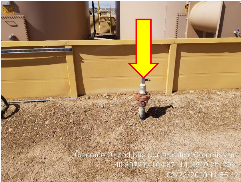
Photo 11 – Unmarked 2” Riser at NE Tank Battery
