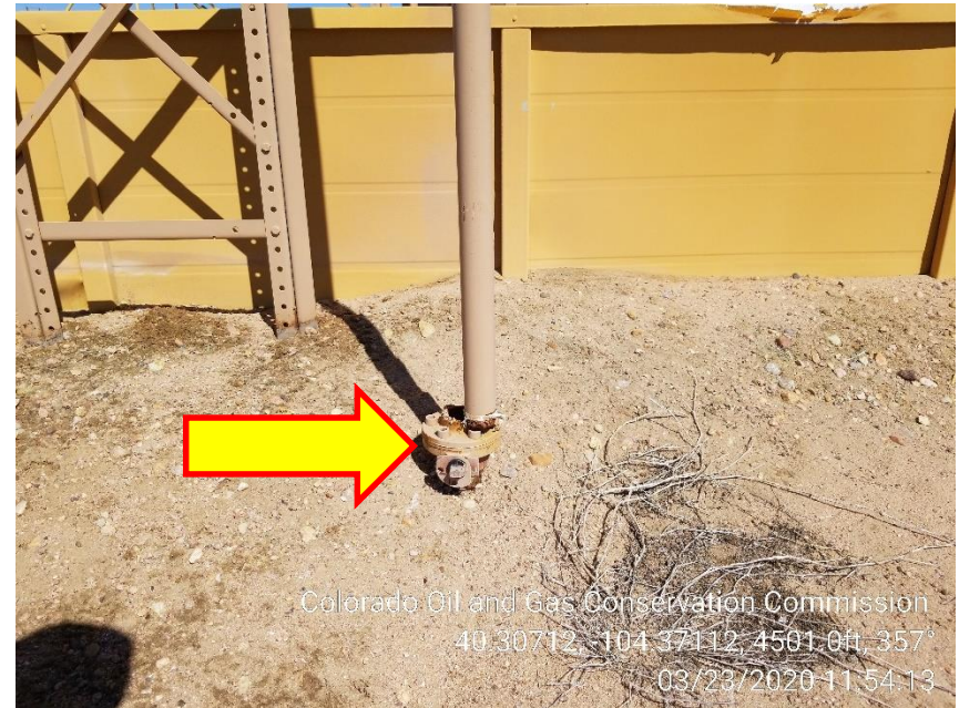
Photo 10 – Unmarked 2" Riser at NE Tank Battery
