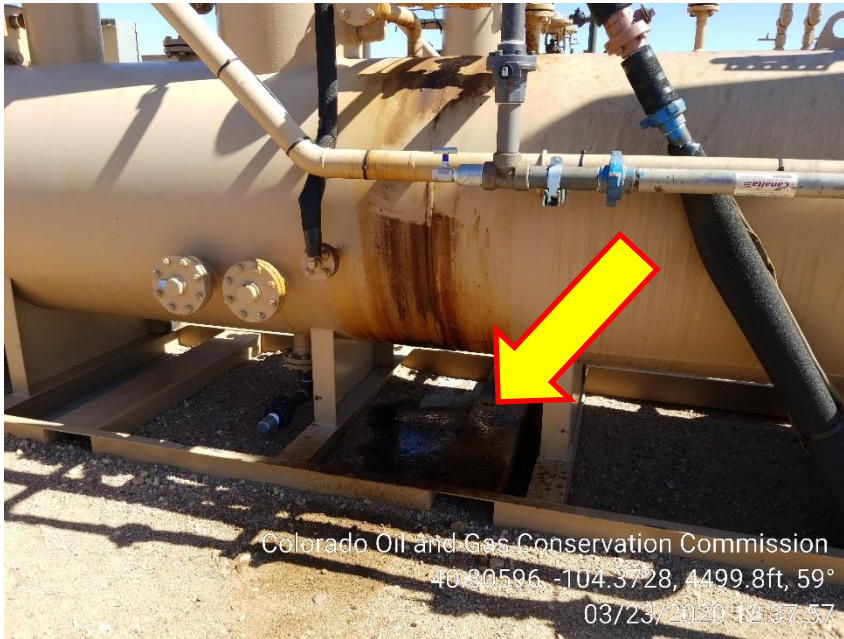
Photo 27 – Stained Soil at West Separator
