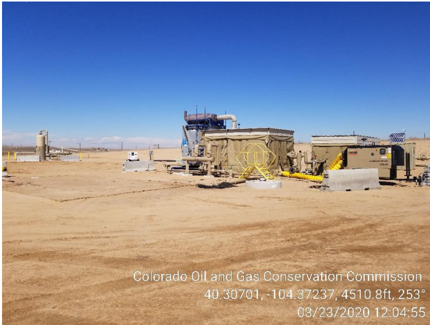
Photo 17 – North Compressor and Gas Meter
