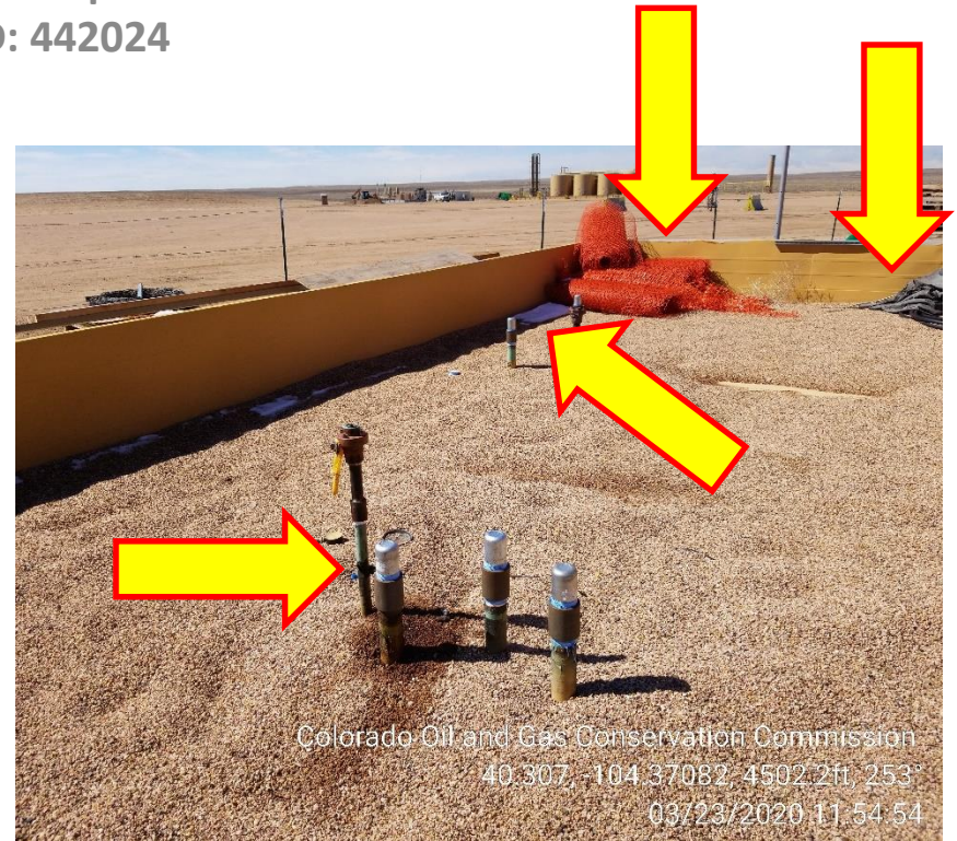
Photo 12 – Unmarked 1” and 2” Risers, Stained Soil and Debris inside the old Separator berm in NE Corner of location.
