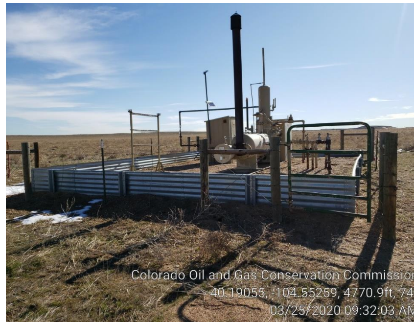
Photo #4 Separator & Meter Run
