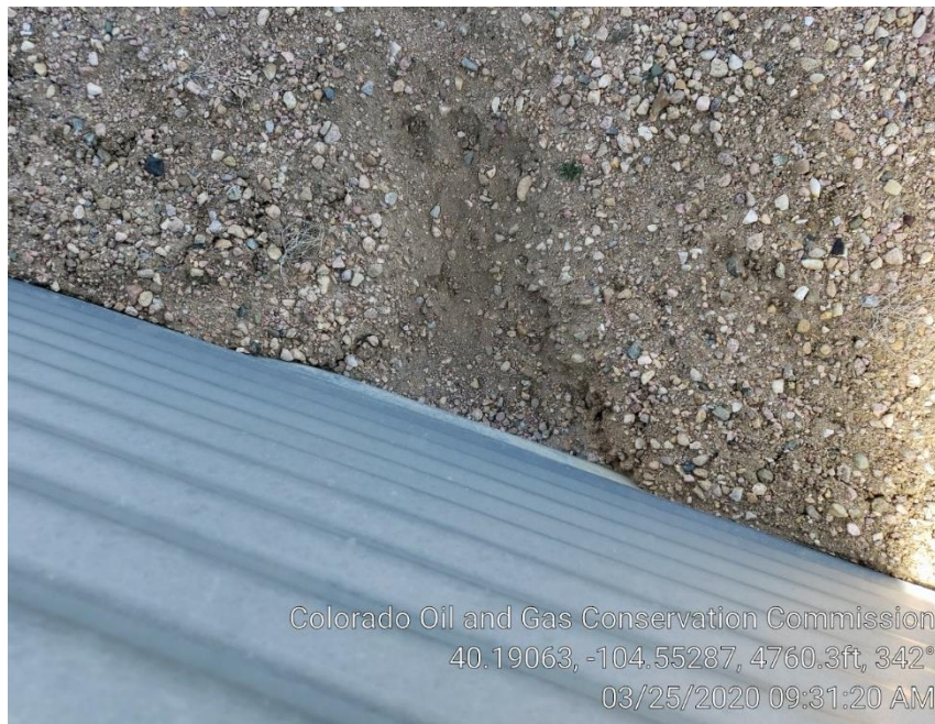
Photo #7 Inadequate berm floor/wall
