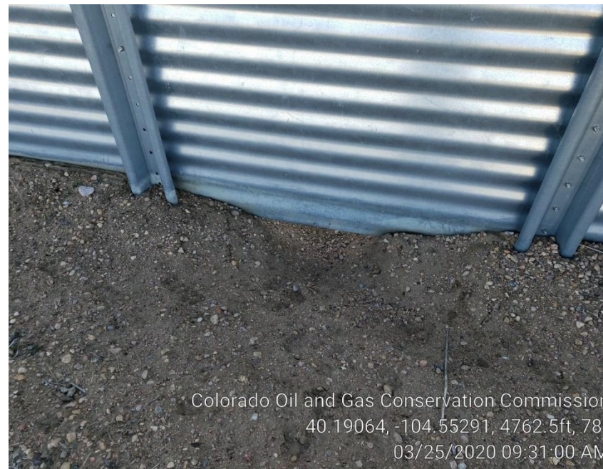
Photo #8 Inadequate berm floor/wall
