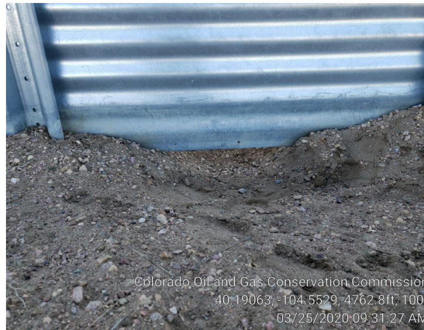
Photo #6 Inadequate berm floor/wall
