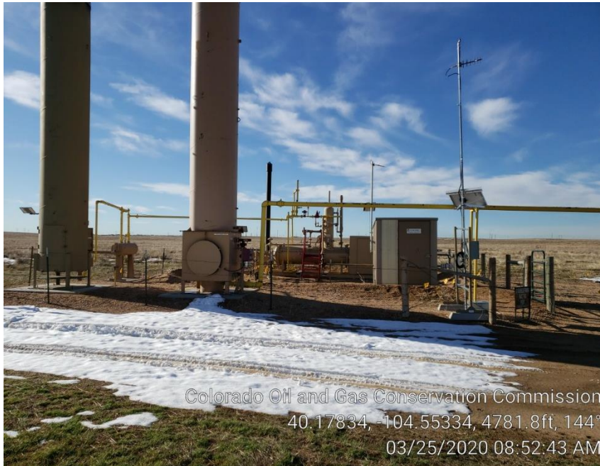
Photo #3 Separator, ECD's & Meter Run
