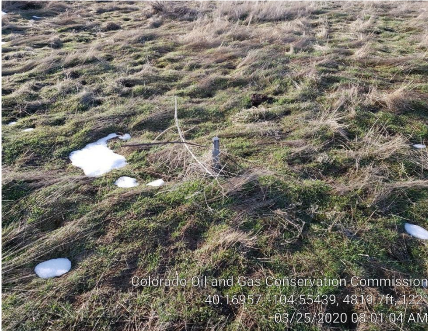
Photo #5 Guy line anchors not marked
