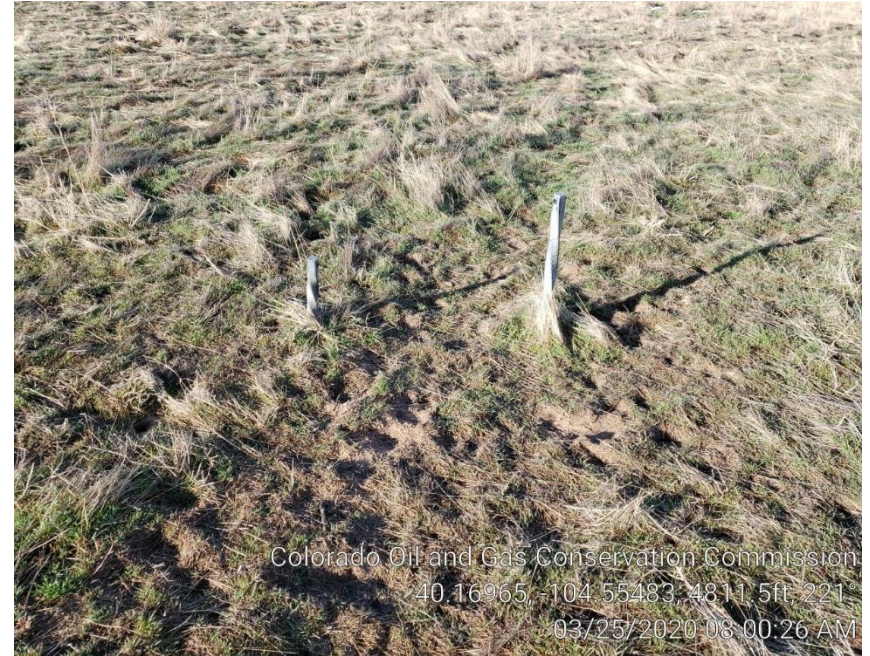
Photo #4 Guy line anchors not marked
