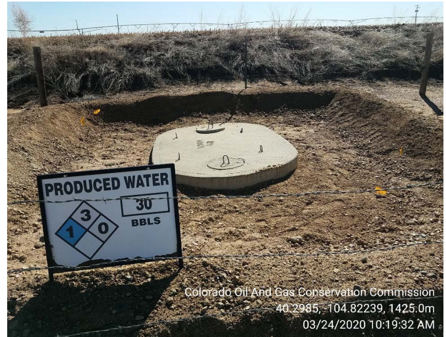
Produced water vault berm on 3/24/2020
