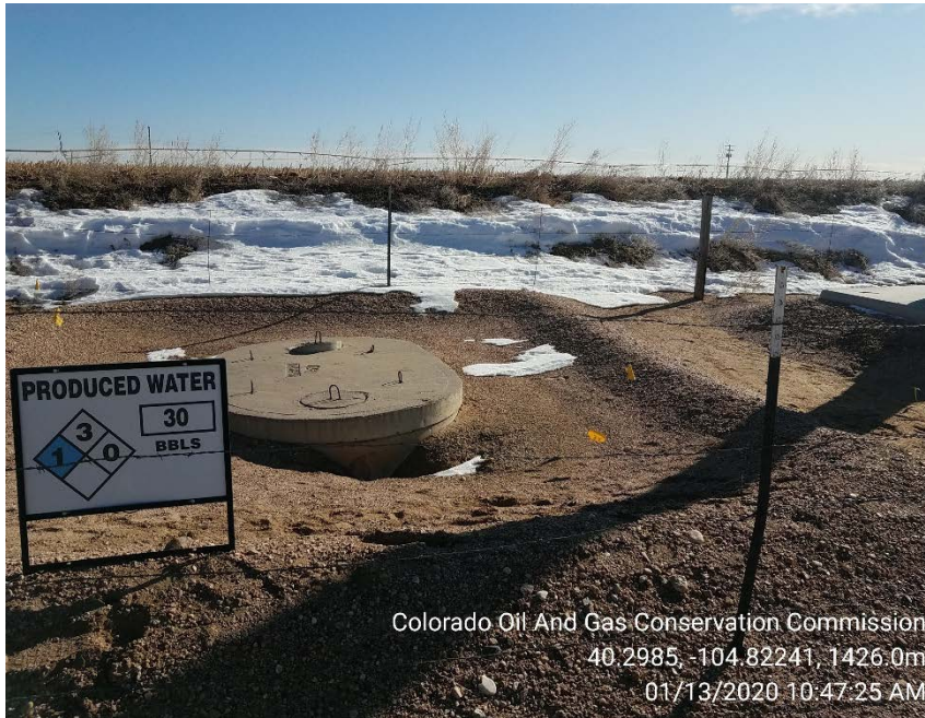
Produced water vault berm on 1/13/2020
