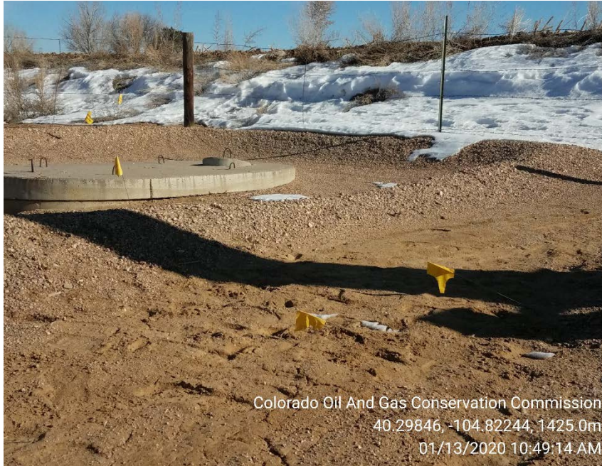
Produced water vault berm on 1/13/2020
