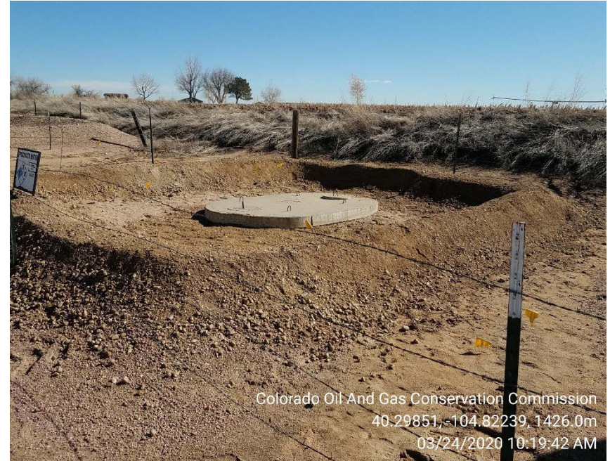
Produced water vault berm on 3/24/2020
