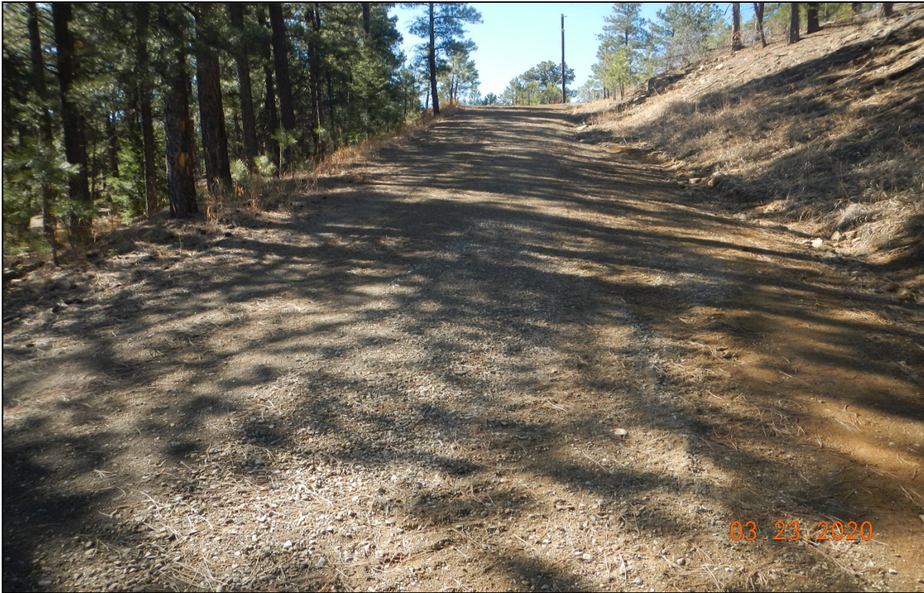
Photo 1. The erosion observed during previous inspection along the pre-existing road has been repaired.
