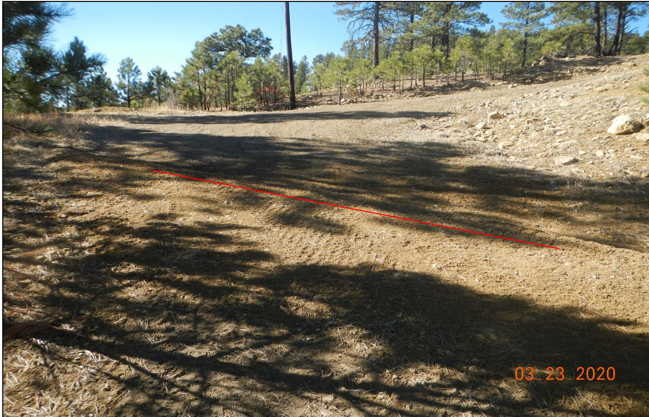
Photo 2. The erosion has been repaired and water bars have been installed along the road. Water bar is installed at red line.
