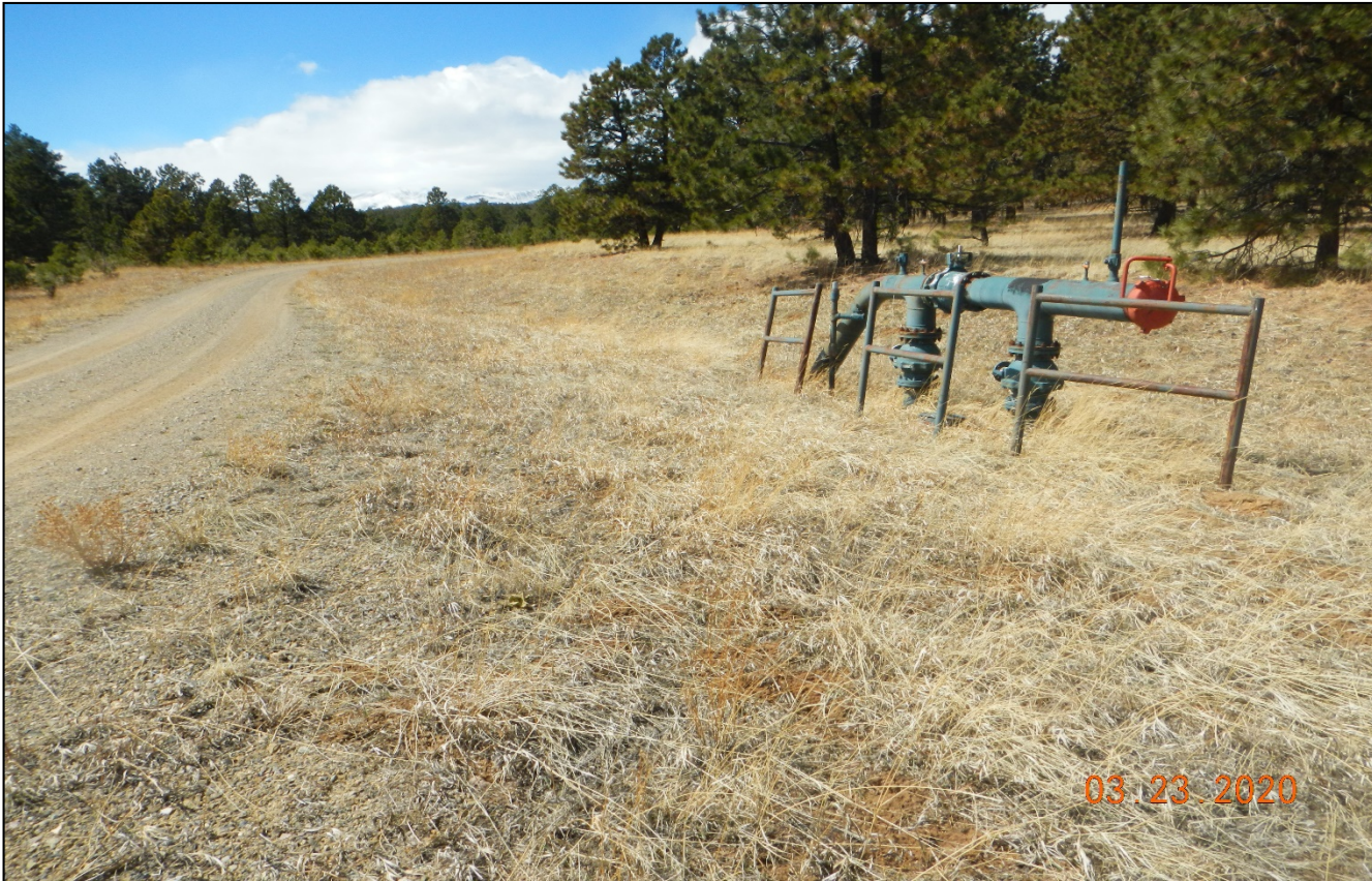
Photo 1. The pig launcher receiver remains along the main access road. No other PR wells remain west along the road. Lat/Long: 37.25975,-104.97719.
