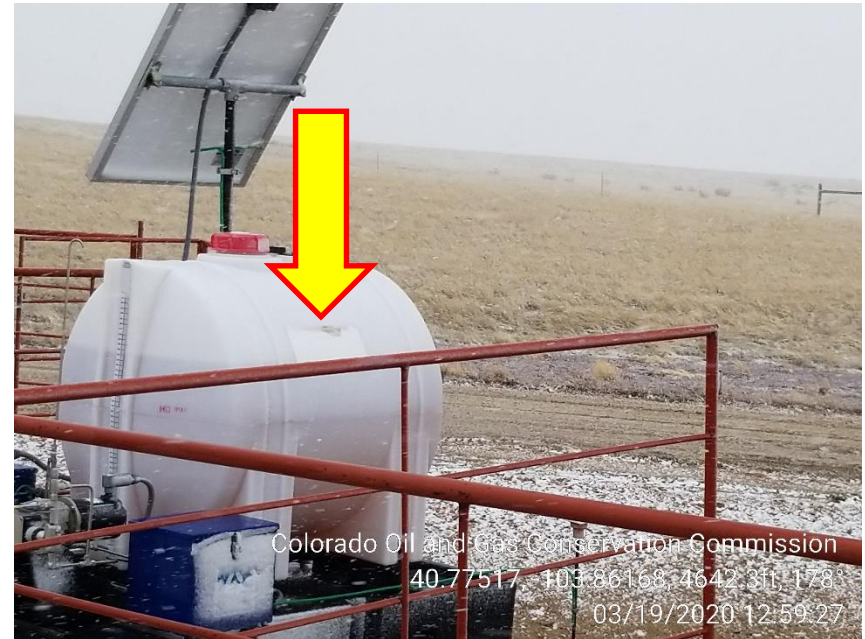
Photo 6 – Chemical Tank label has faded
