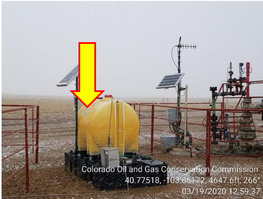
Photo 5 – Chemical Tank label has faded
