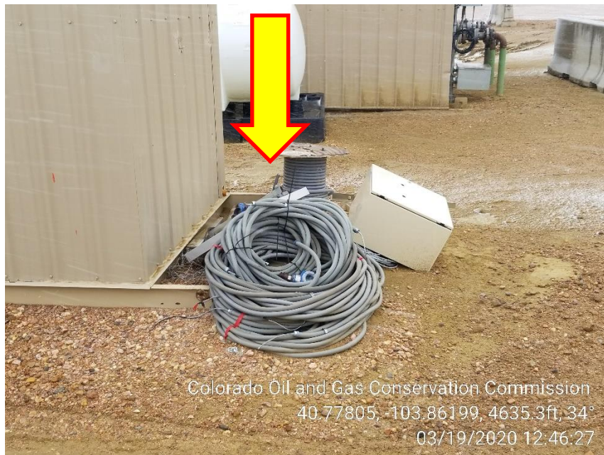
Photo 9 – Unused Automation wires at South Gas Lift Meter Houses
