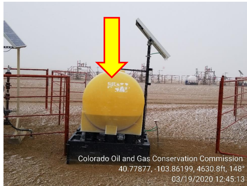
Photo 8 – Chemical Label has faded at West Wellheads
