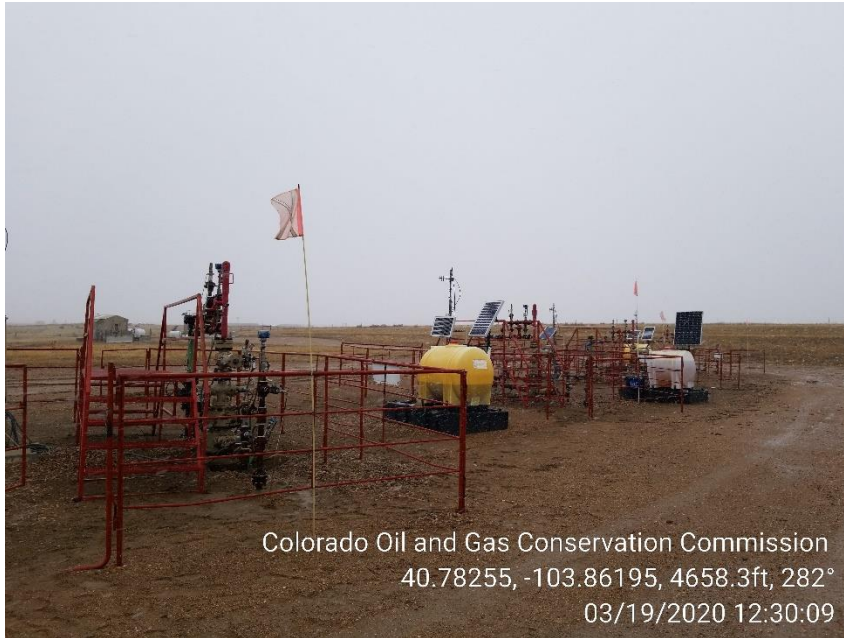
Photo 3 – Wellheads
