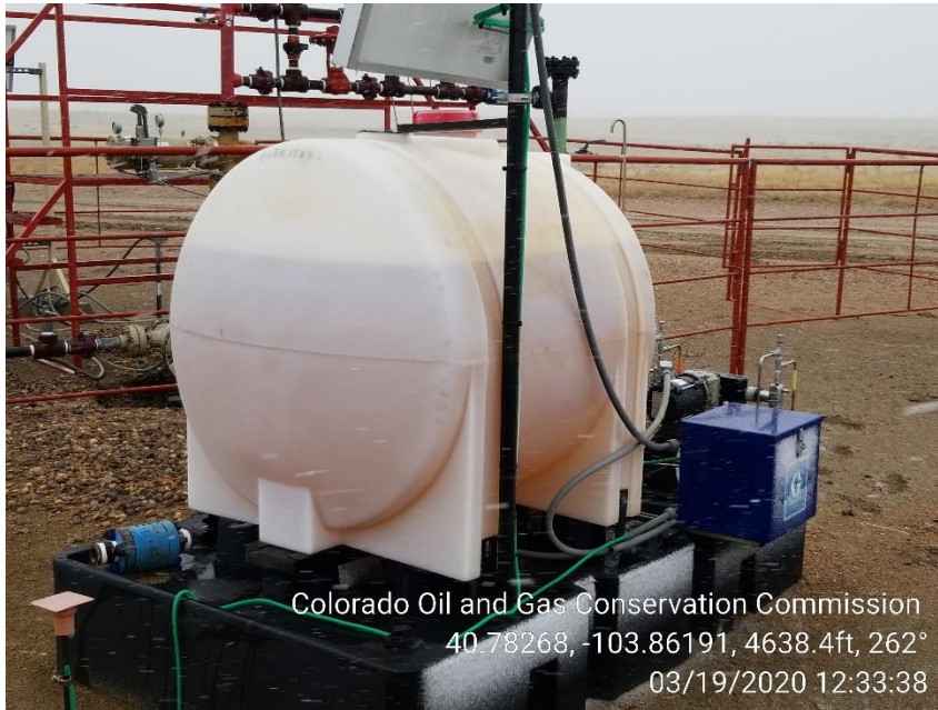
Photo 7 – Chemical Tank missing Labels
