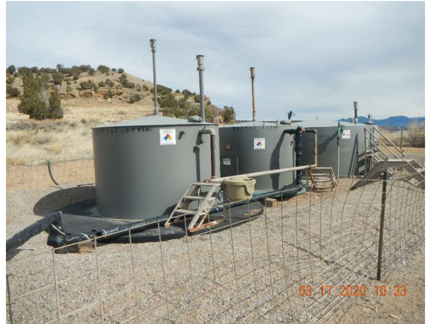
Tank battery looking east, 2 80 bbl Produced Water steel ASTs and a 200 bbl Condensate steel AST.
