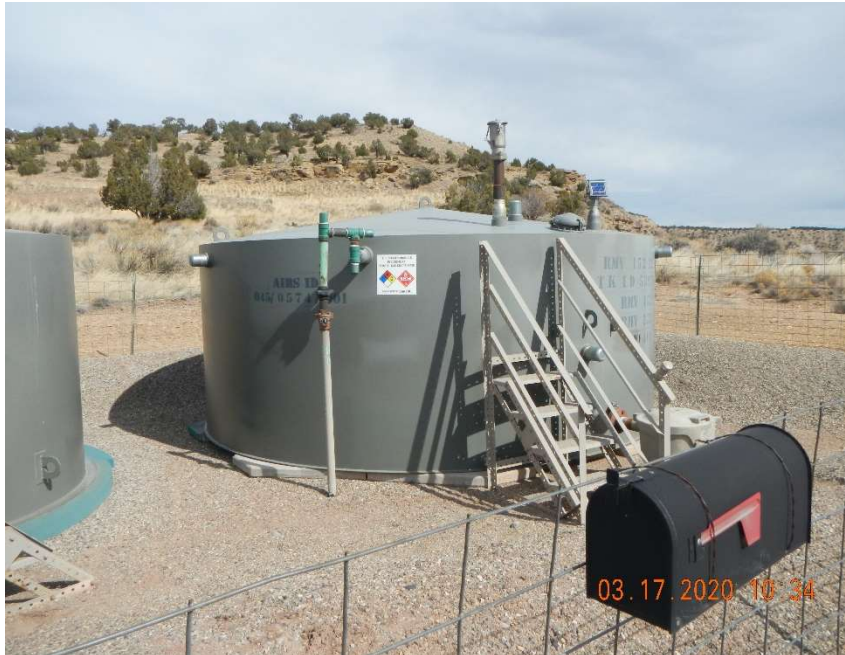
200 bbl Condensate steel AST.
