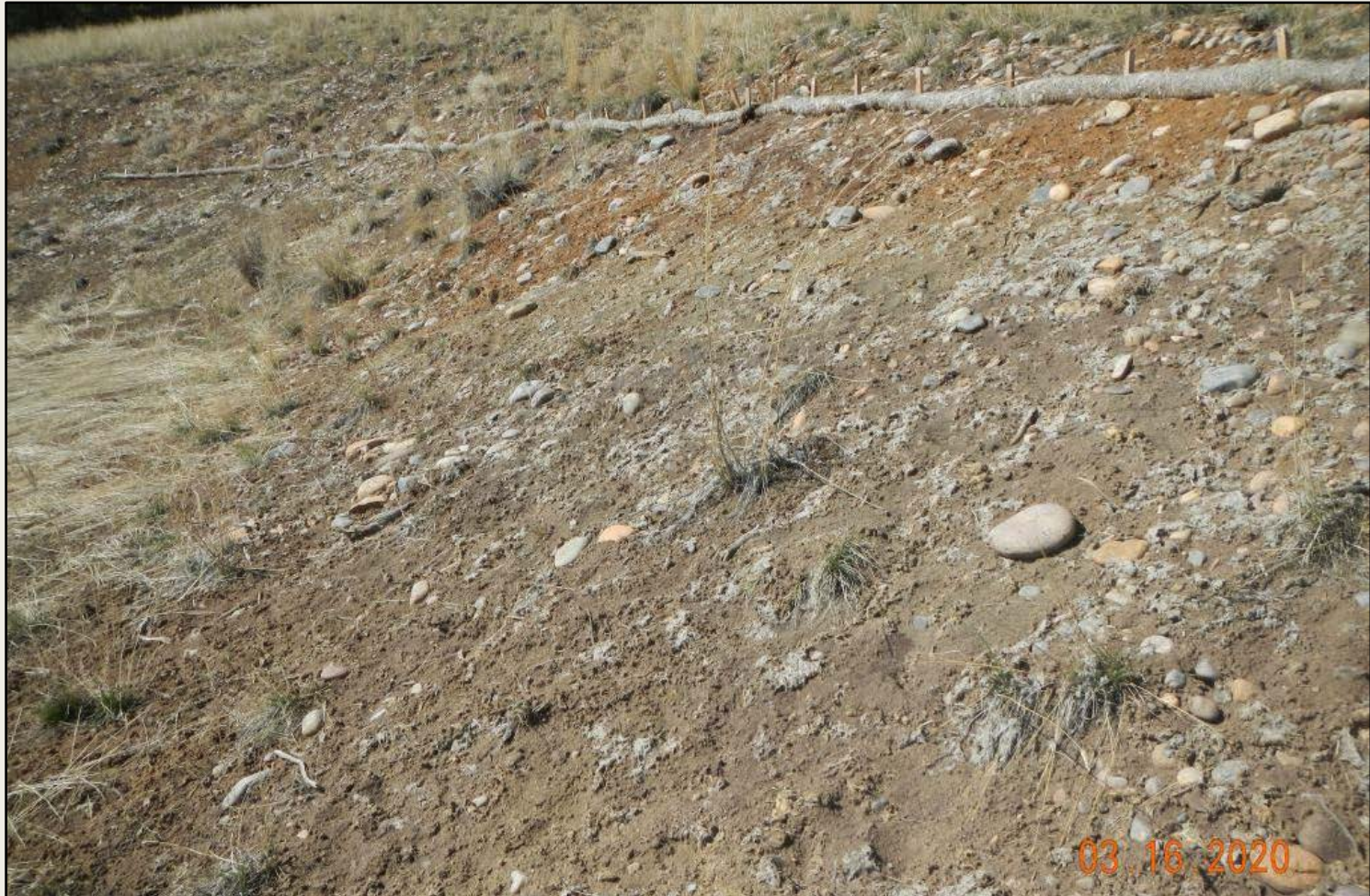
Photo 3. View of the northwestern cut-slope. Hydromulch and wattle on slope. Revegetation progressing in portions and remains sparse in other portions. Needs to be monitored during the 2020 growing season and if not progressing then additional measures will be needed.
