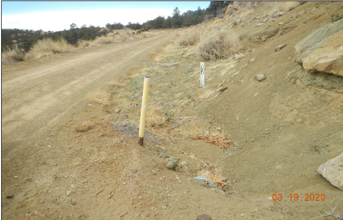
Photo 1. The culvert along the main lease road ascending the hill to the location is filled in with sediment.
