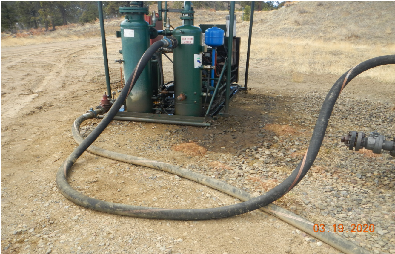
Photo 3. There is oil stained soil around the engine skid that needs to be cleaned up.
