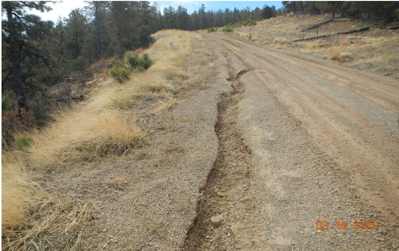
Photo 6. There is erosion occurring down the road as it ascends to the top of the hill. Approx. Lat/Long:37.12287,-104.95893.
