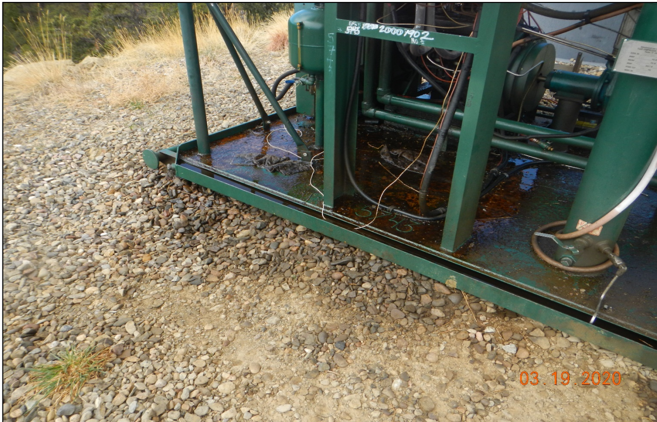
Photo 5. There is oil on the engine skid and on soil that needs to be cleaned up.
