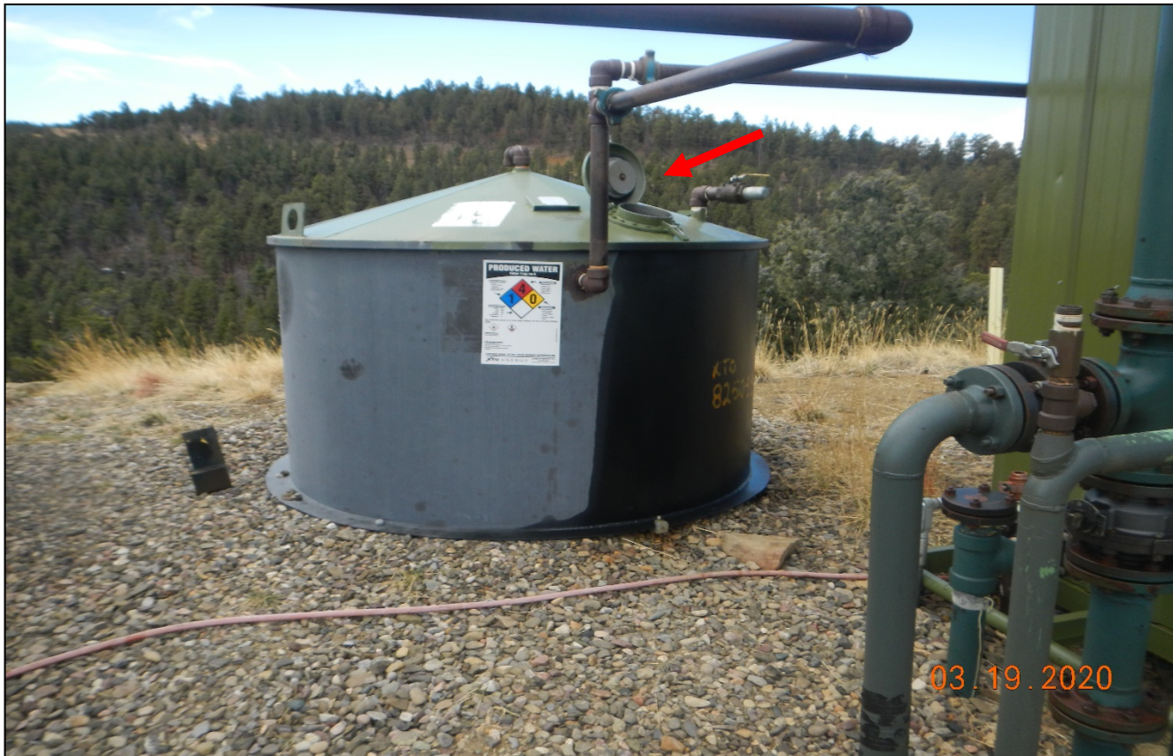
Photo 4. There is staining coming from the tank. The lid is open and appear which appears to have spilled out of.
