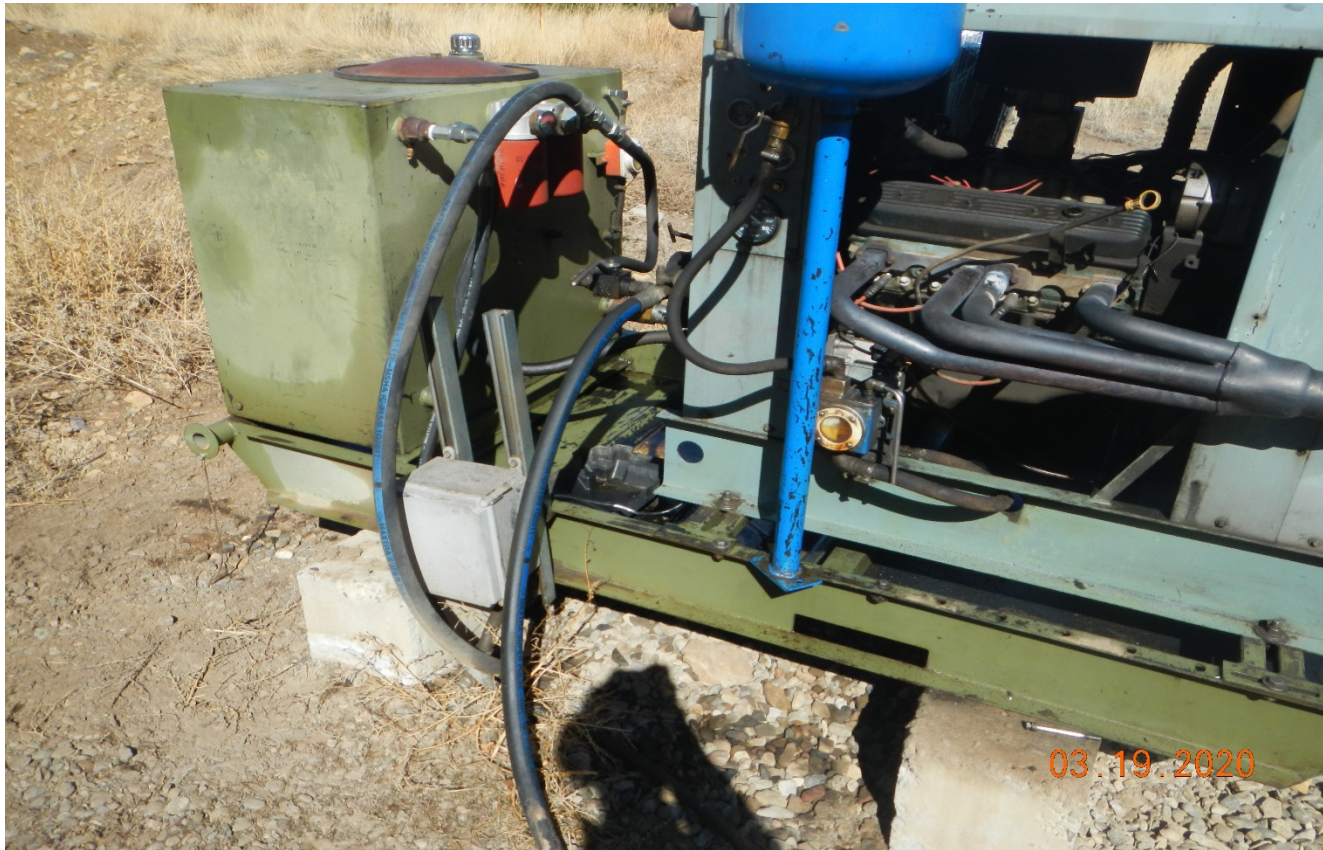
Photo 6. The oil on the engine skid has been cleaned up since previous inspection.
