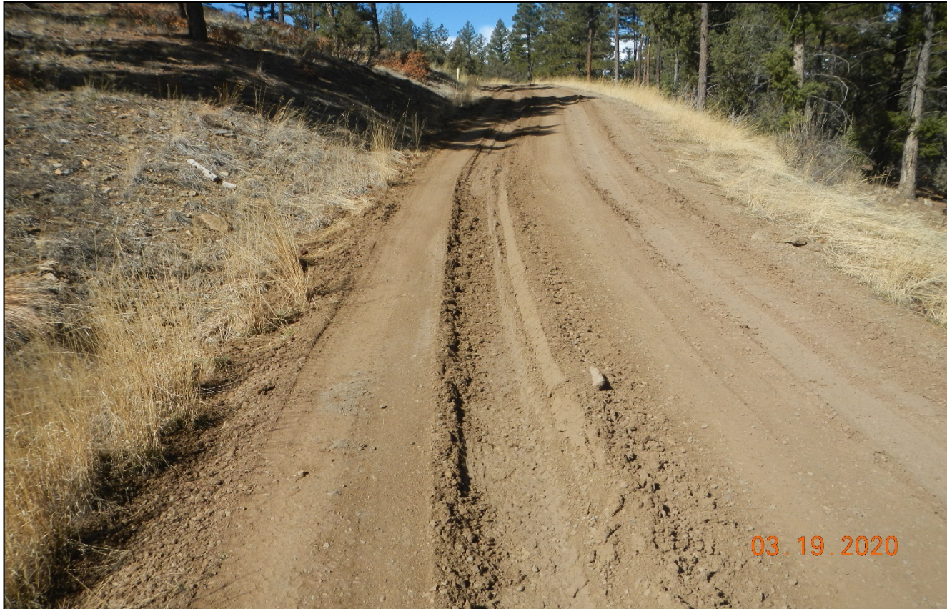
Photo 1. Facing southwest along the access road. There are vehicle ruts along the road. The road needs to be graded and maintained.
