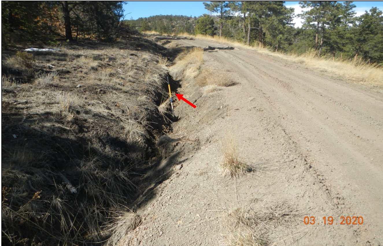
Photo 3. There is erosion occurring on the side of the access road that needs to be repaired and stabilized. Arrow points to 4.5 ft. shovel for scale.
