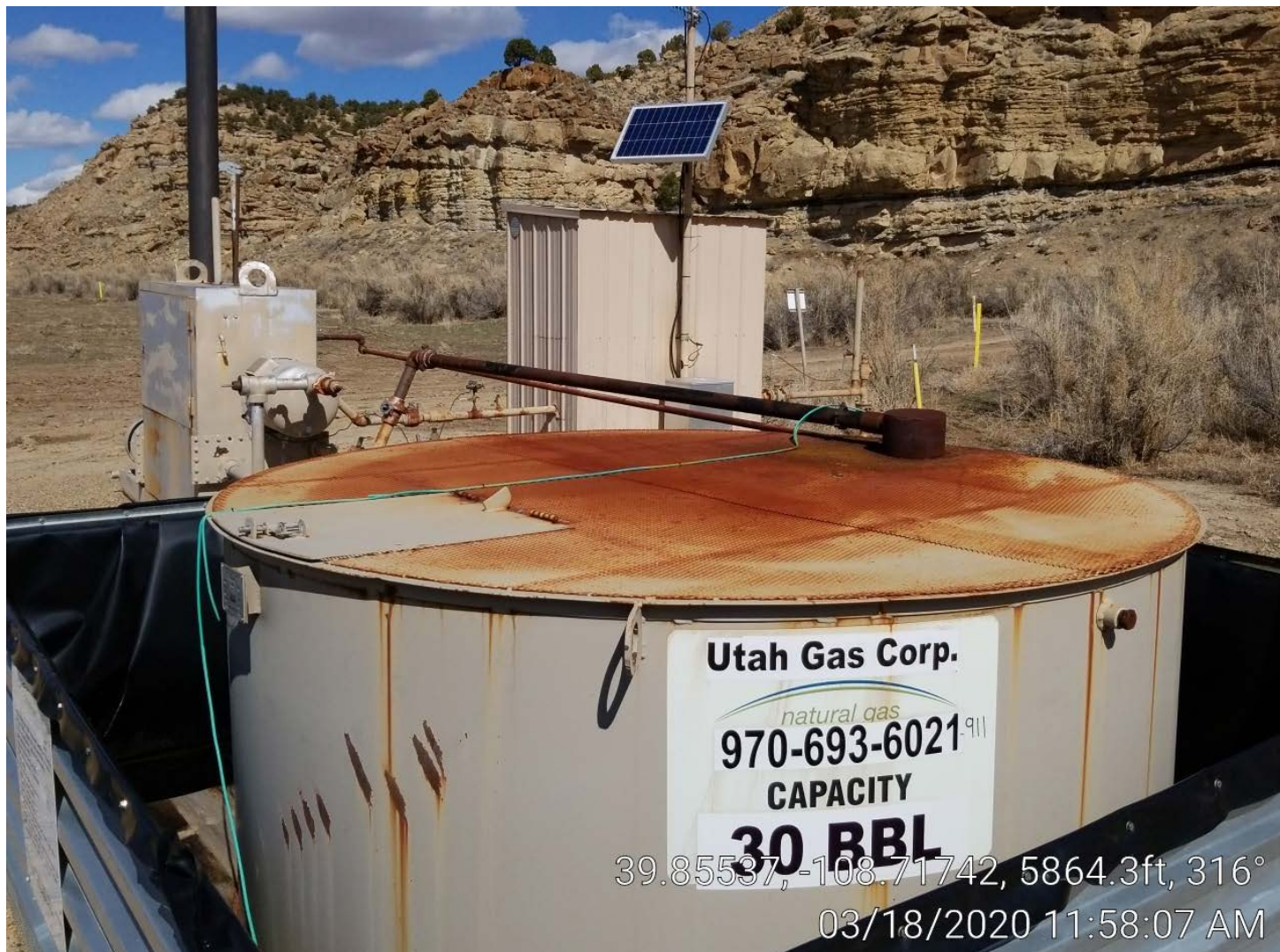
Photo 2. Tank, meter building, and separator.
