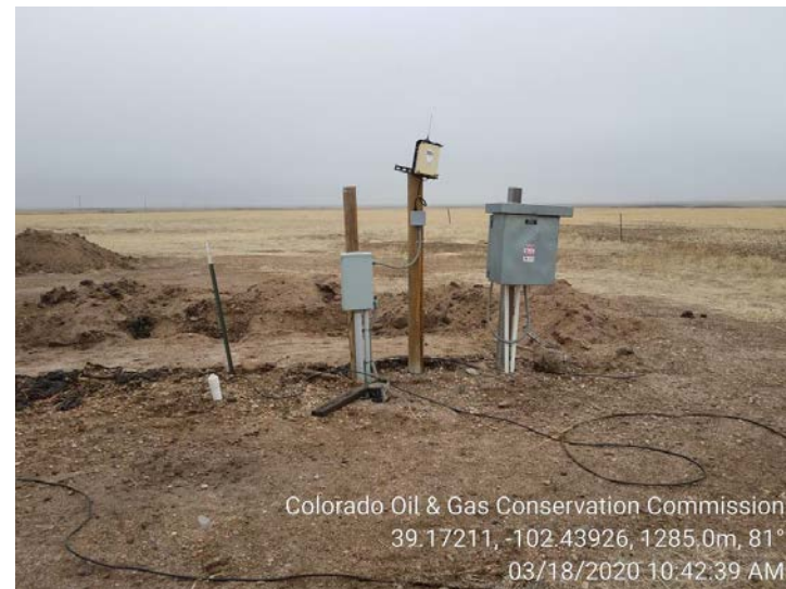
8. Electric panel and Cathodic Rectifier
