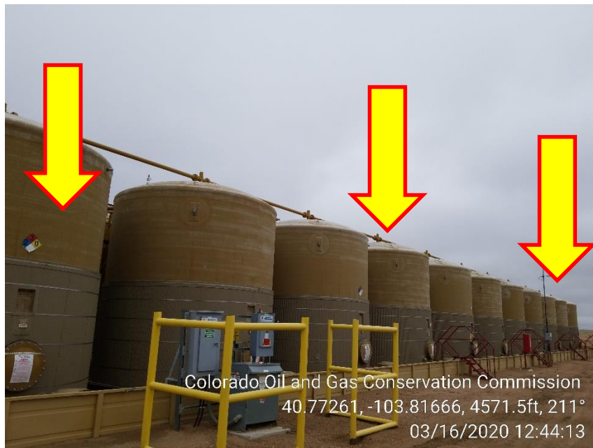
Photo 7 – Southside Water Tanks, Content and Capacity missing on all Tanks
