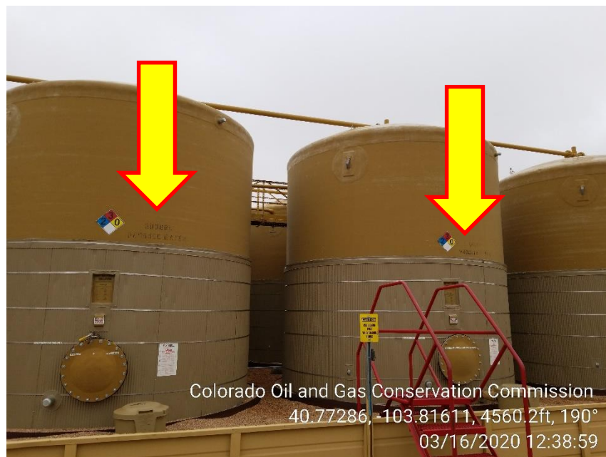
Photo 5 – Northside Water Tanks, Content and Capacity fading, no longer visible
