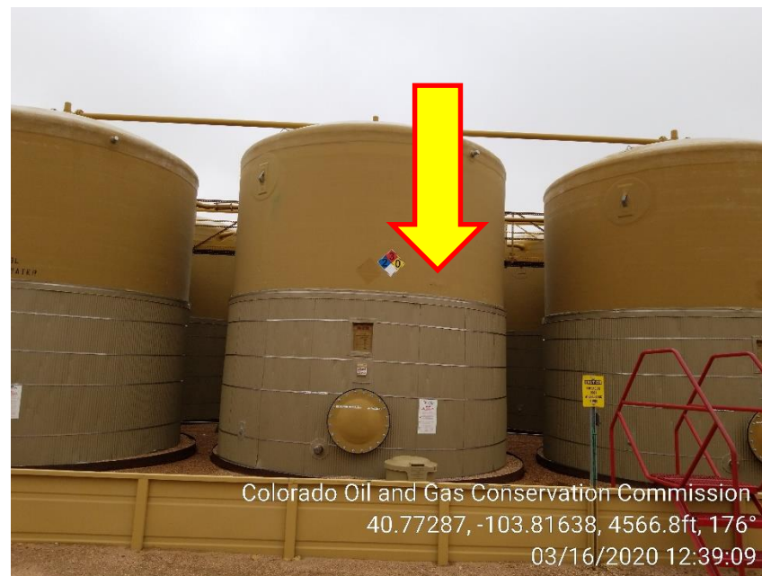
Photo 6 – Northside Water Tanks, Content and Capacity missing
