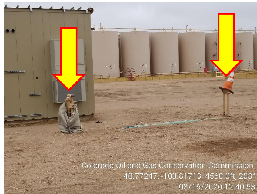
Photo 8 – Unmarked Risers at NW shed
