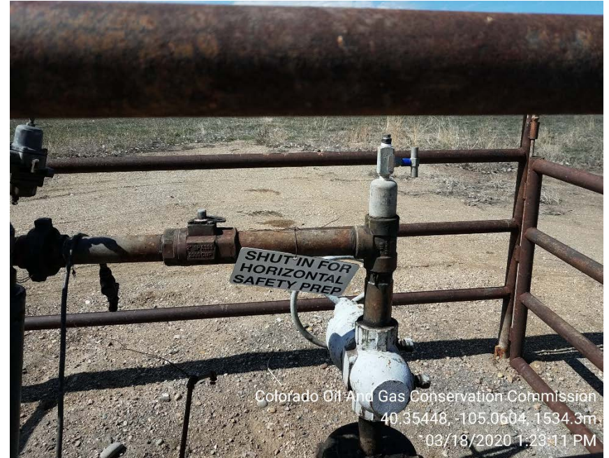
HZ safety prep sign
