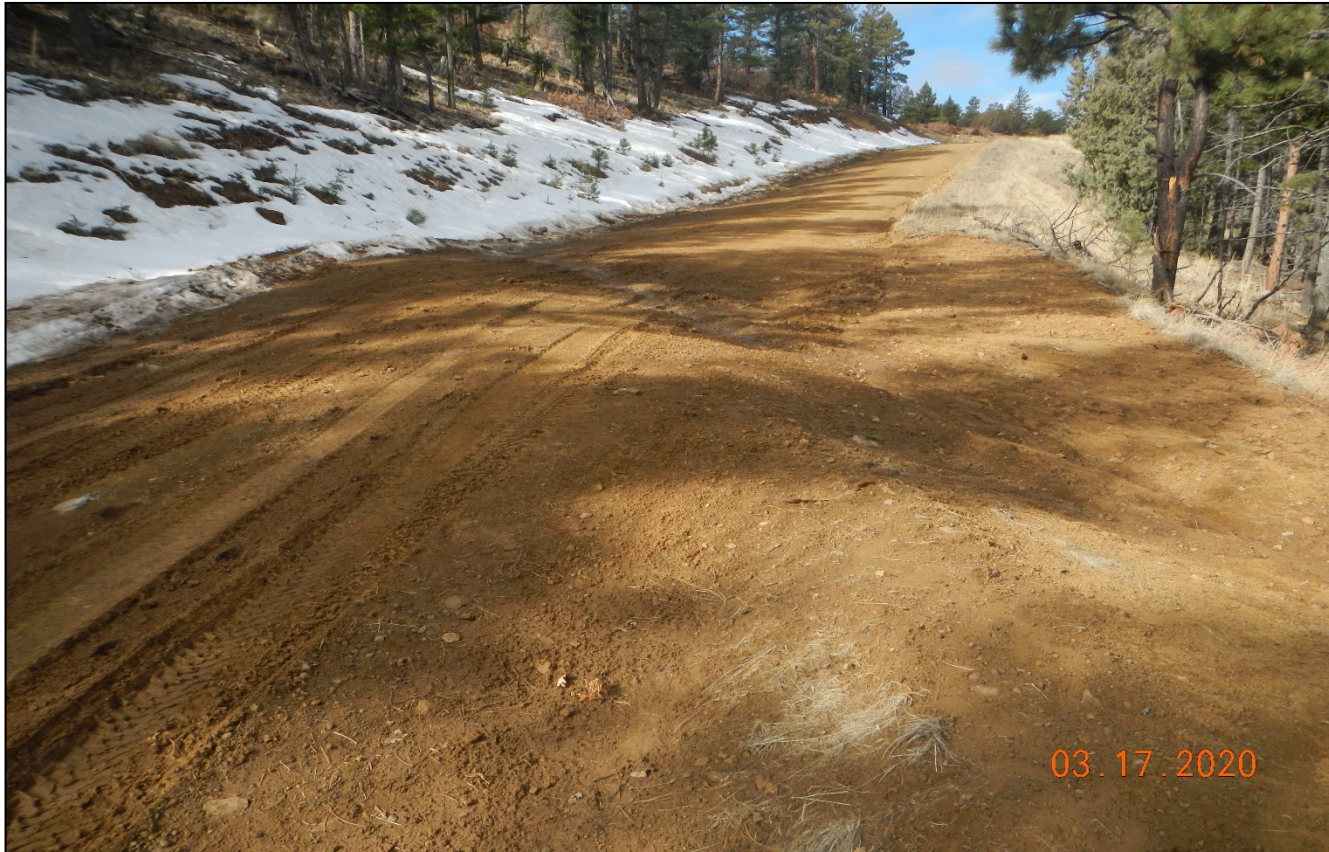
Photo 2. There are several water bars installed along the main lease road.
