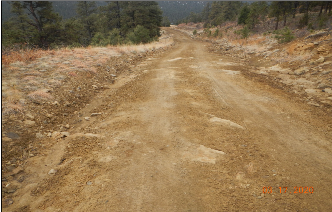
Photo 1. Facing south along the access road. The road has been graded.
