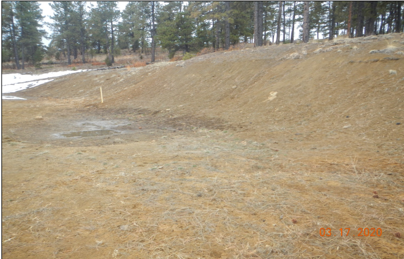
Photo 4. Facing southwest toward the cut slope. This area is bare of vegetation and needs to be monitored and reseeded as needed for revegetation.
