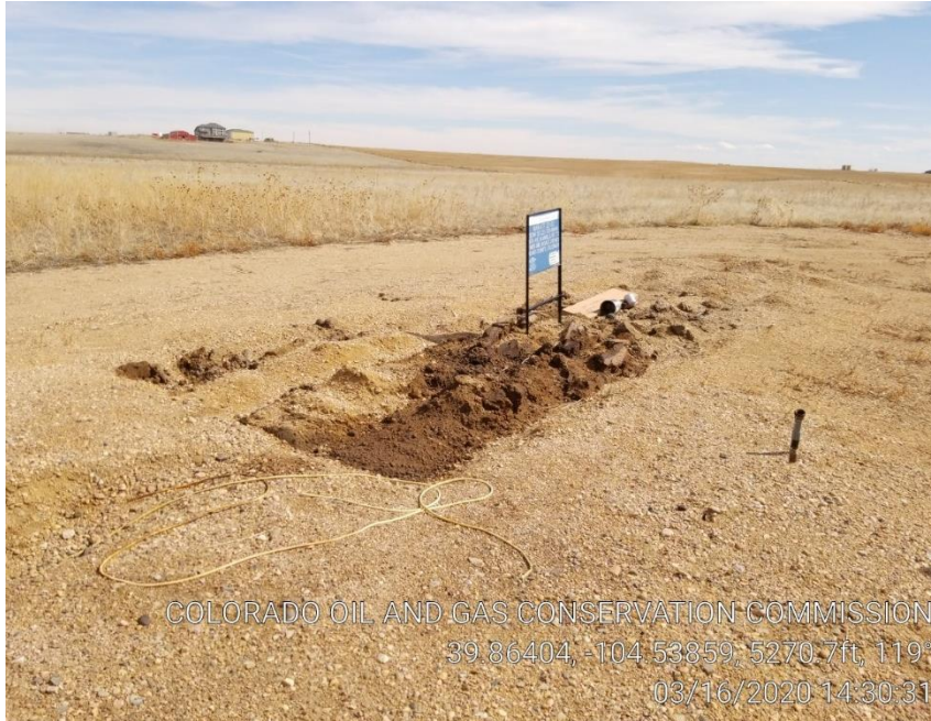
Pic 1 stained soil, riser with no LOTO, trash.
