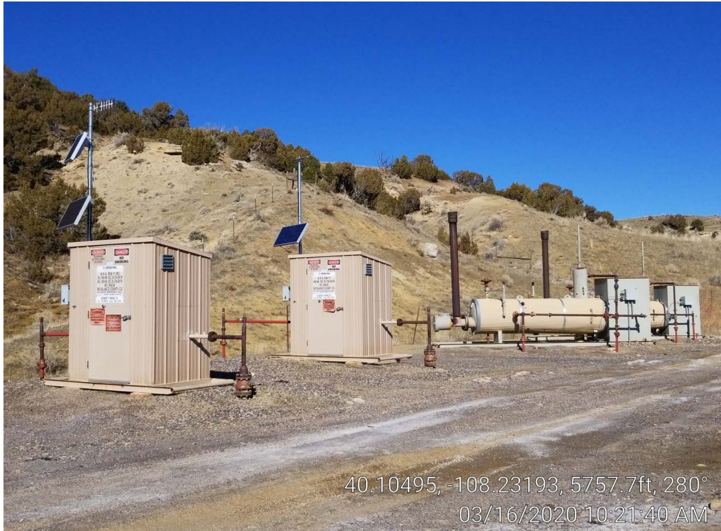
Photo 3. Meter buildings & separators.
