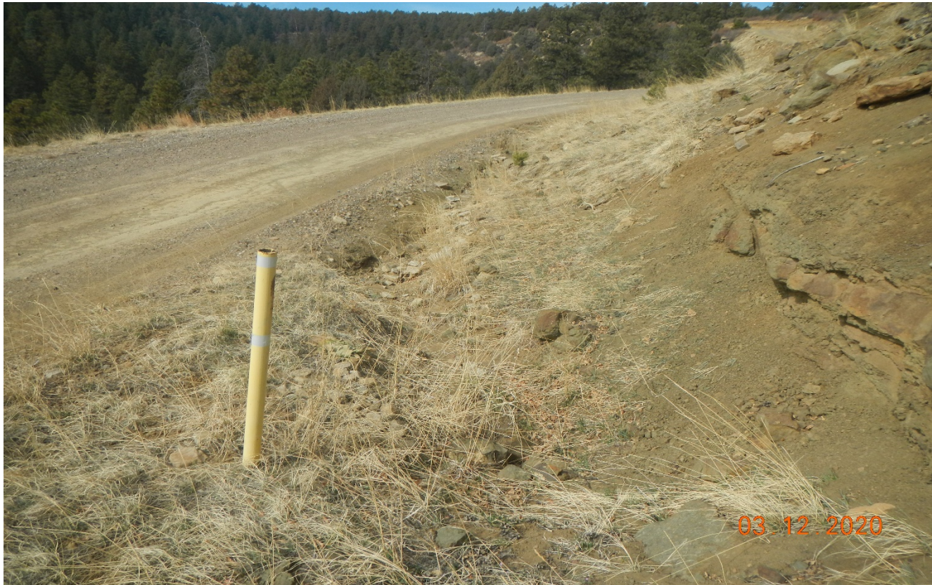
Photo 9. This culvert has filled in with sediment along main access road toward the compressor station.
