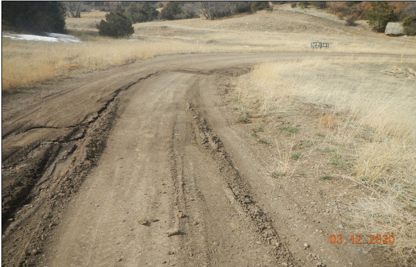
Photo 3. Stormwater is flowing down the road and not properly diverted. Lat/Long:37.05382,-104.87658.
