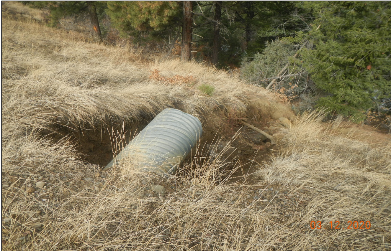
Photo 2. The culvert outlet is causing erosion at Lat/Long:37.05382,-104.86860.
