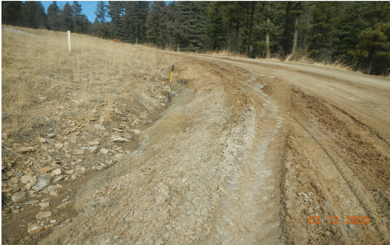
Photo 8. There is erosion on the side of the road at Lat/Long:37.05713,-104.87836.
