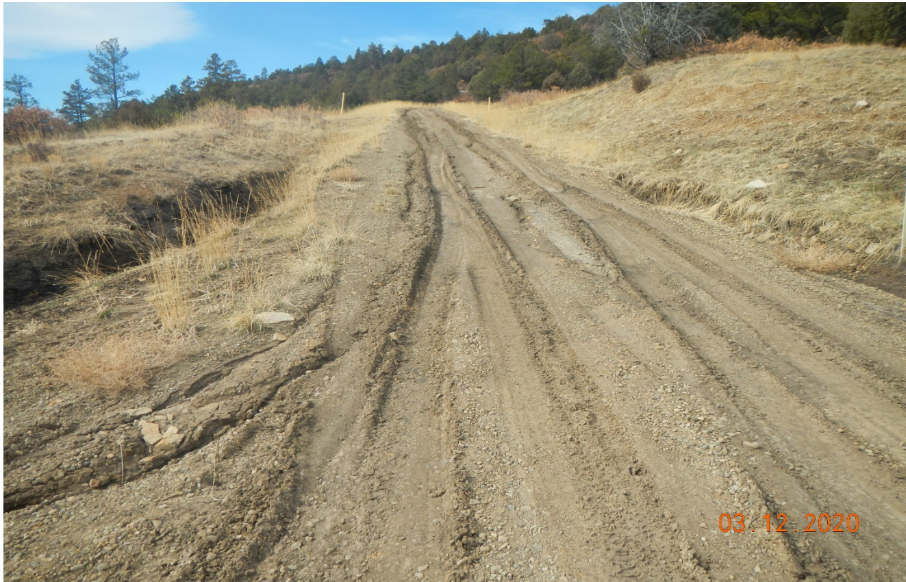
Photo 5. There is vehicle rutting along the access road to the location..
