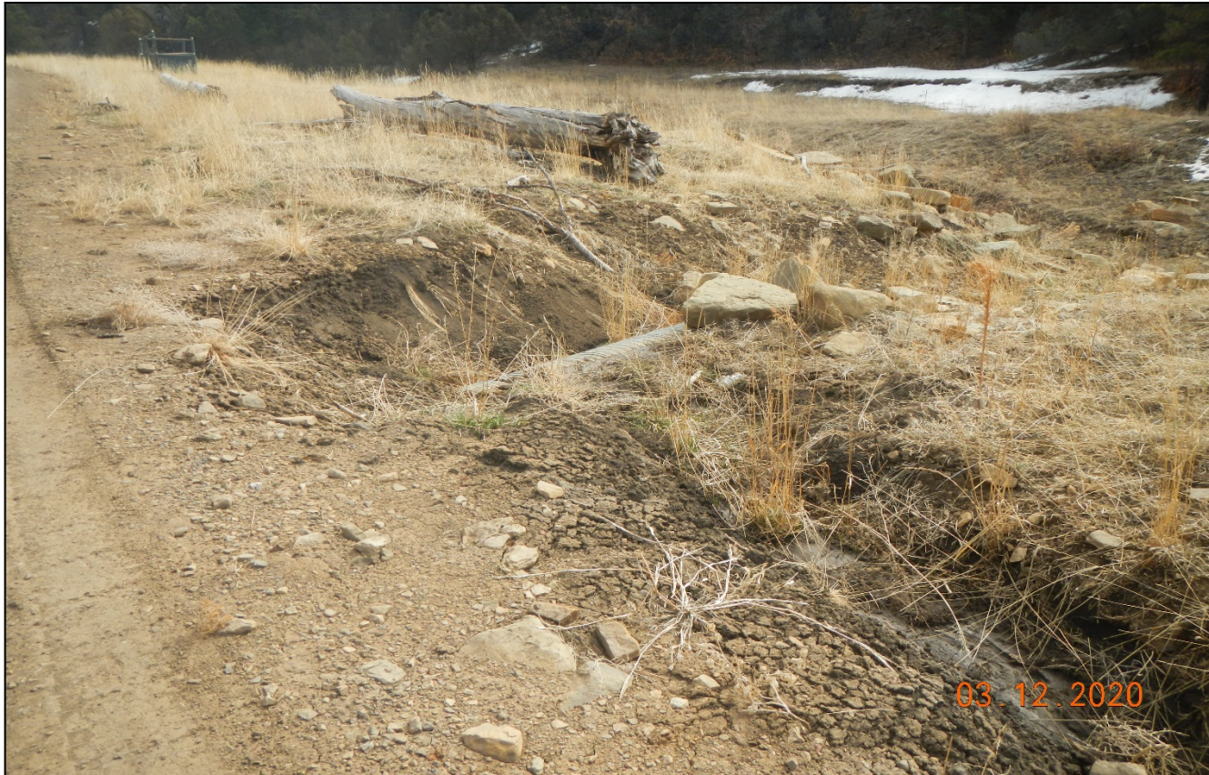
Photo 4. The is erosion occurring at the culvert outlet at Lat/Long:37.05059,-104.87625.
