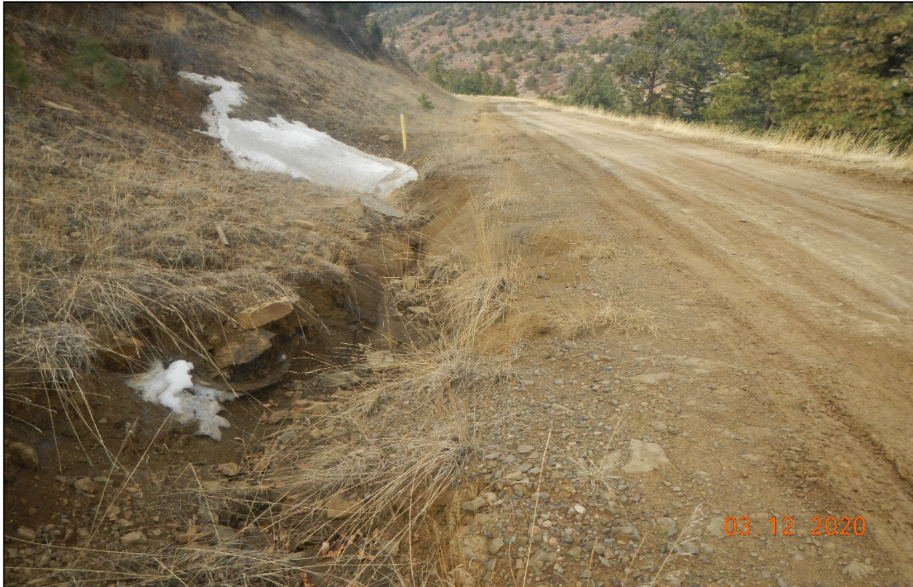
Photo 1. There is erosion occurring at this culvert inlet along the main road at Lat/Long:37.05382,-104.86860. It is unknown because of snow cover if culvert inlet is filled in.
