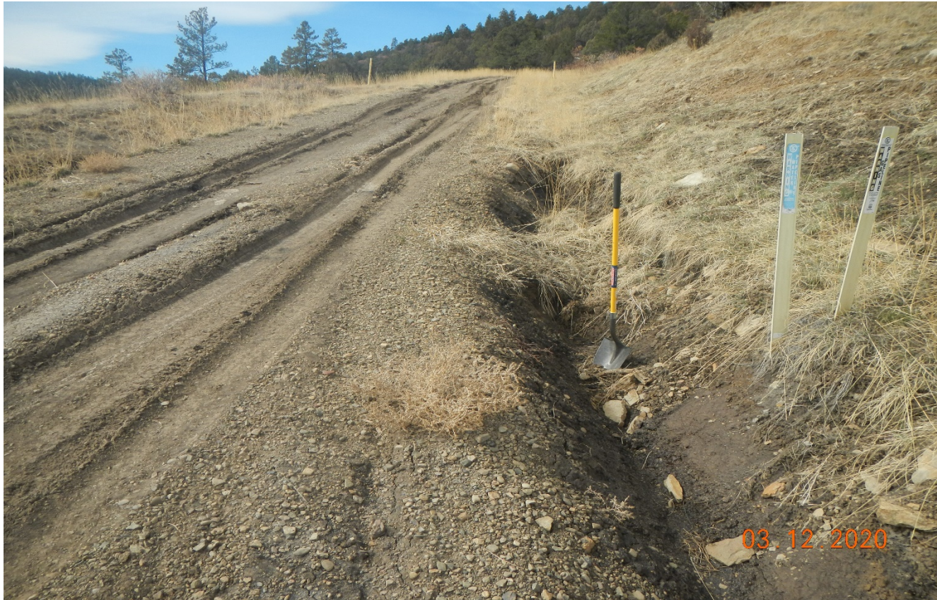
Photo 6. There is erosion occurring along the sides of the access road.
