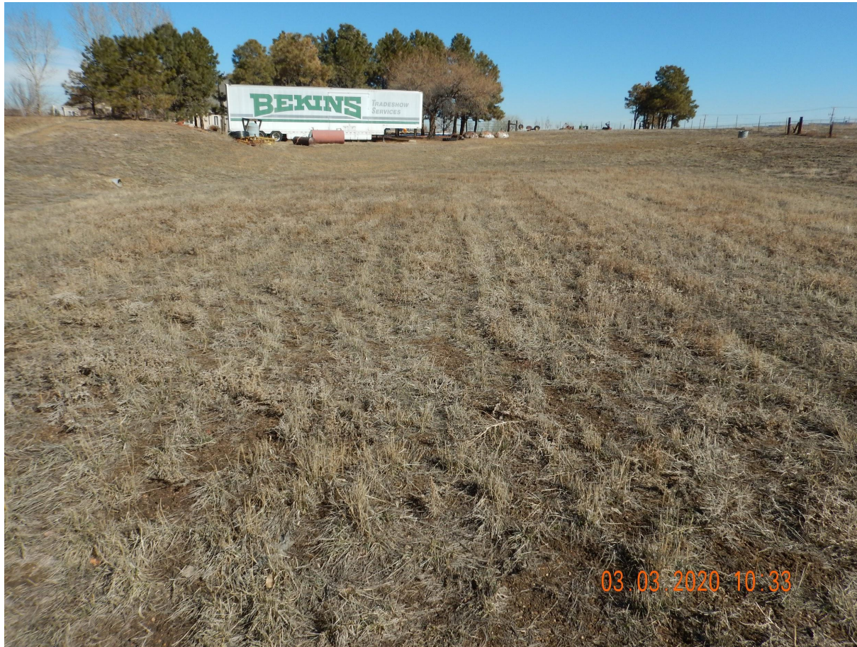
Photo 1. Photo taken from the well and tank battery location, facing North. All equipment has been removed. No noxious weeds or stormwater erosion issues observed.
