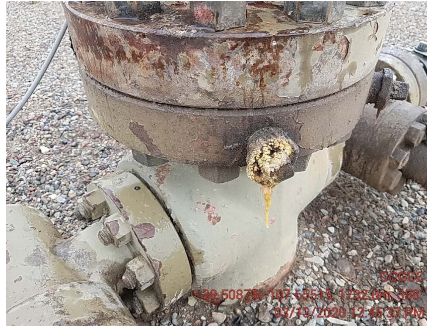
Leaking wellhead
