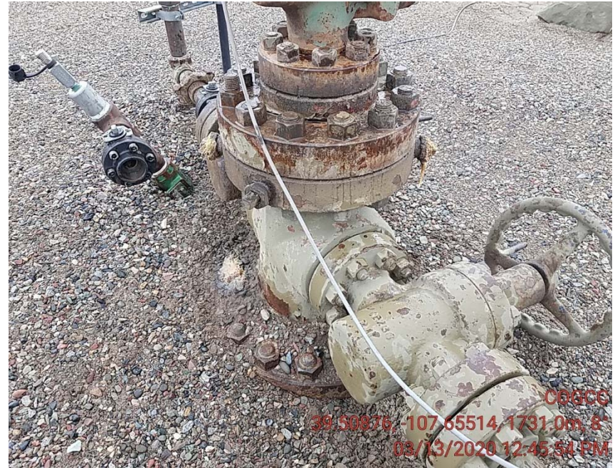
Leaking wellhead
