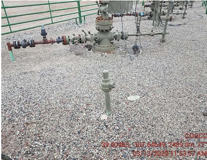
Unmarked flow line
