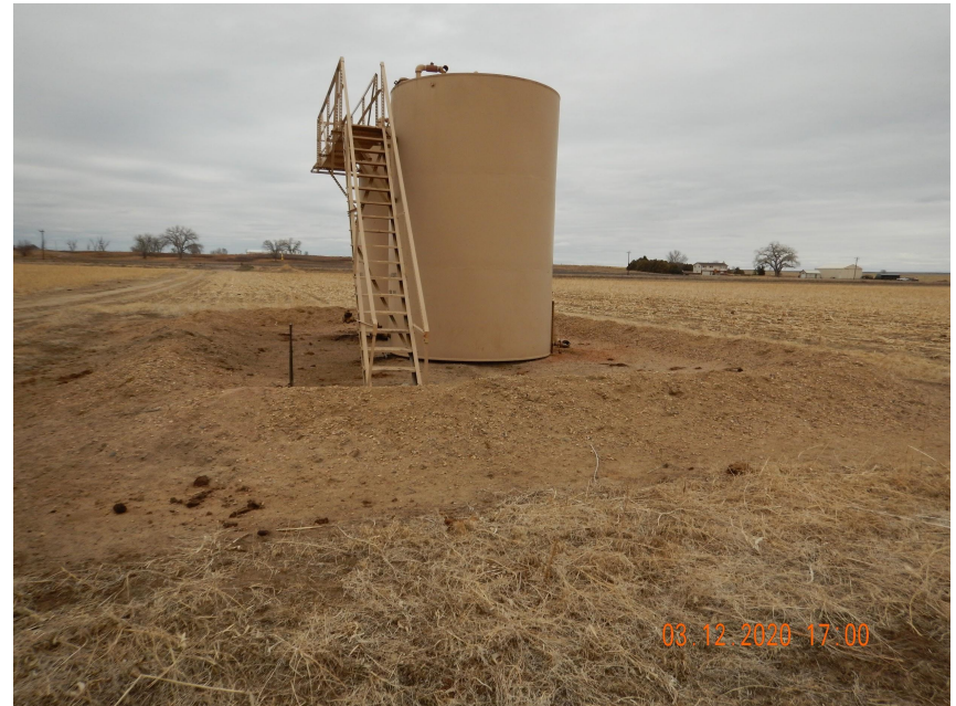
Photo 2. Photo taken from the eastern location, facing North. Photo illustrates Operator has failed to remove all equipment from location. All equipment should have been removed by 5/13/2019. Also, all final reclamation activities should have been conducted by 5/13/2019 due to the location within cropland.
