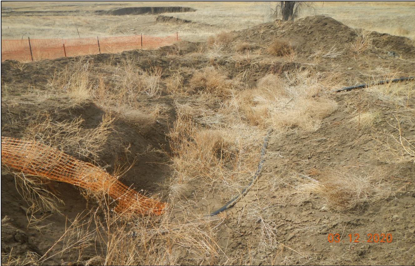
Photo 2. The open excavation area is about 4 ft. deep. Weeds have grown in this area during previous growing season.
