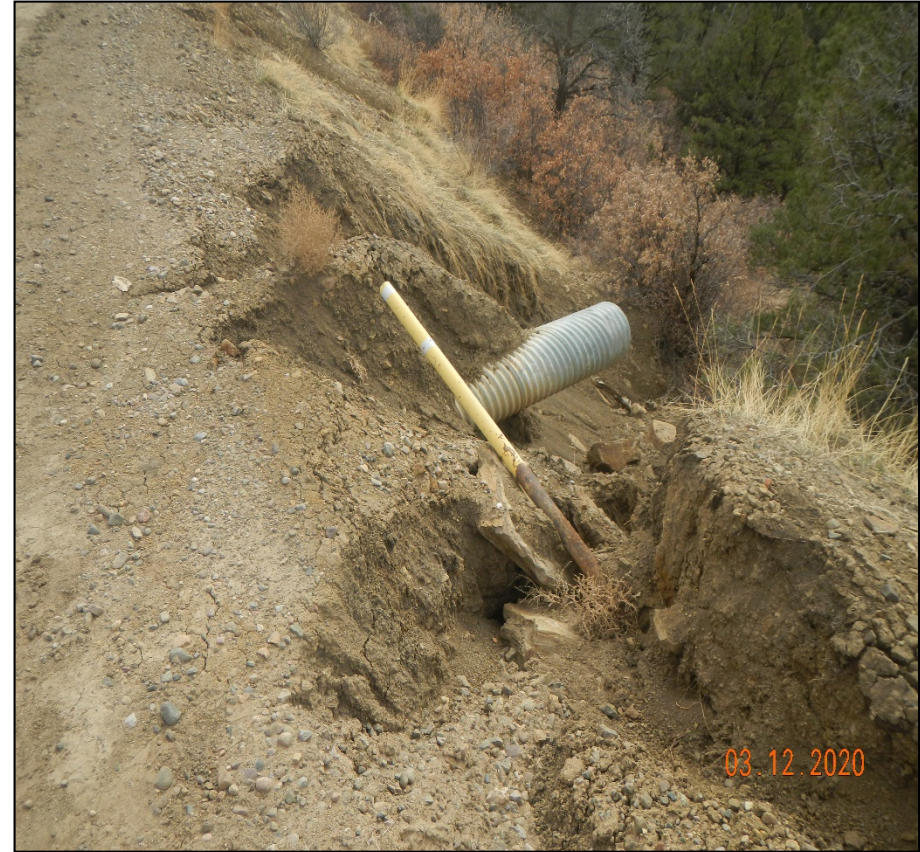
Photo 7. Photo 5. Stormwater runoff from the road is causing erosion near this culvert at Lat/Long:37.05297,-104.82619. There is no outlet protection installed at the culvert outlet.
