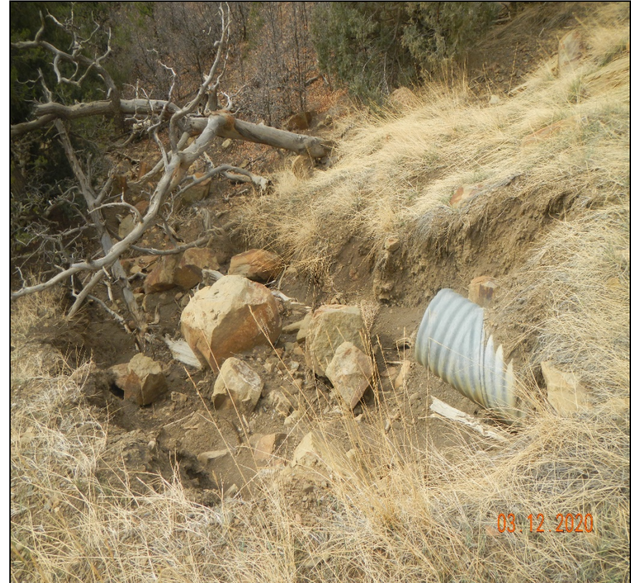
Photo 6. The above photos of the culvert inlet and outlet were taken at Lat/Long:37.05354,-104.82491. The inlet culvert has filled in with sediment and the outlet culvert is causing erosion.
