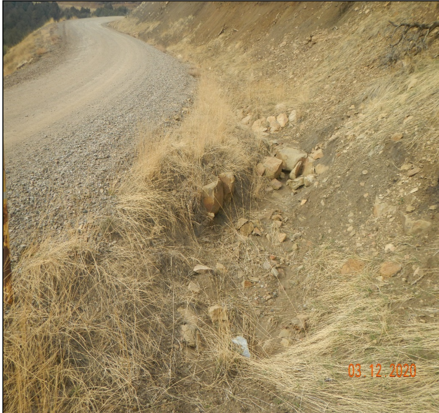
Photo 6. The above photos of the culvert inlet and outlet were taken at Lat/Long:37.05354,-104.82491. The inlet culvert has filled in with sediment and the outlet culvert is causing erosion.
