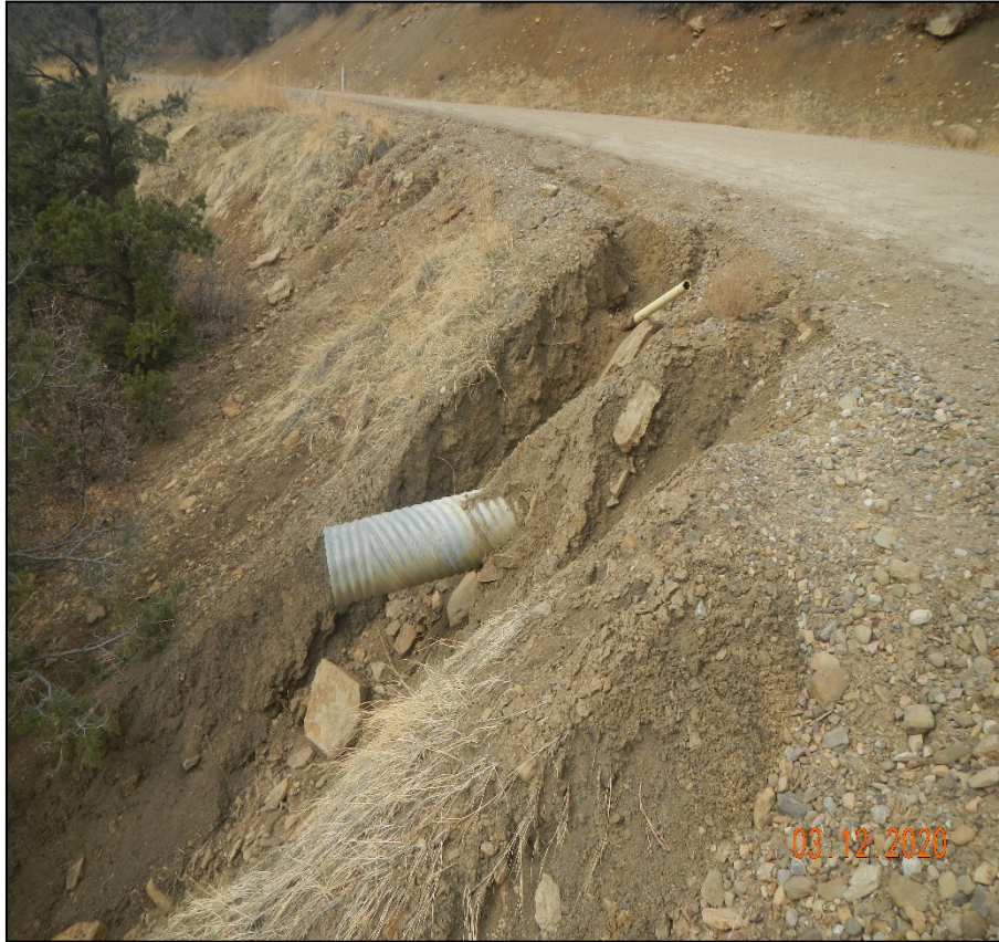
Photo 7. Photo 5. Stormwater runoff from the road is causing erosion near this culvert at Lat/Long:37.05297,-104.82619. There is no outlet protection installed at the culvert outlet.
